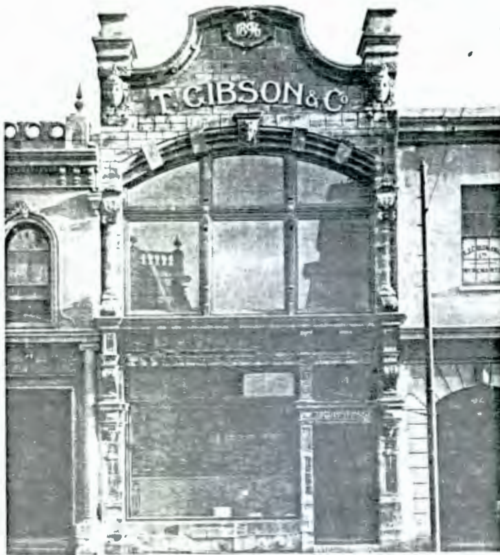
Gibson & Co, Long St. 1904. De Witt. Undoubtedly the best example of Art Nouveau architecture still left in Cape Town. The façade is entirely of terracotta, with pilasters supporting a decorated frieze, and relief panels bearing the name of the firm. Heavy floral trusses support the next tier of columns above which shields support a wide arch spanning the building; the parapet consists of a wavy moulding against the skyline, flanked by two Medusa heads. Originally there was gilded lettering telling the firm's name and date, which shone against the rose-pink walls.
