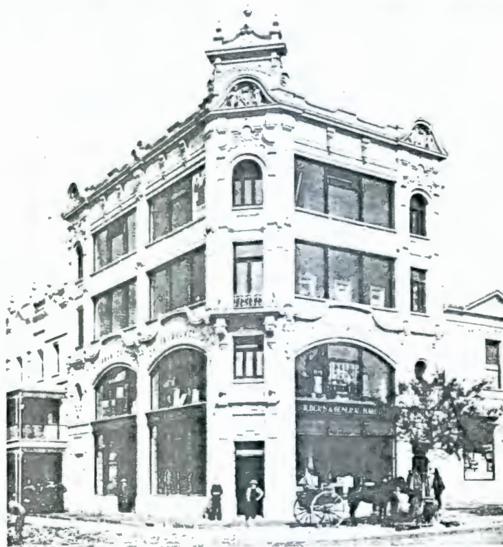
Chubb & Maxwell, Wale/ Loop St. 1905. De Witt. In spite of the frills of plasterwork this building was an innovation, and was built upon a framework of steel supplied by Dorman Long. The large plate-glass windows set into this framework give to the design a simplicity quite apart from their functional value. Later, the building was destroyed by fire.
