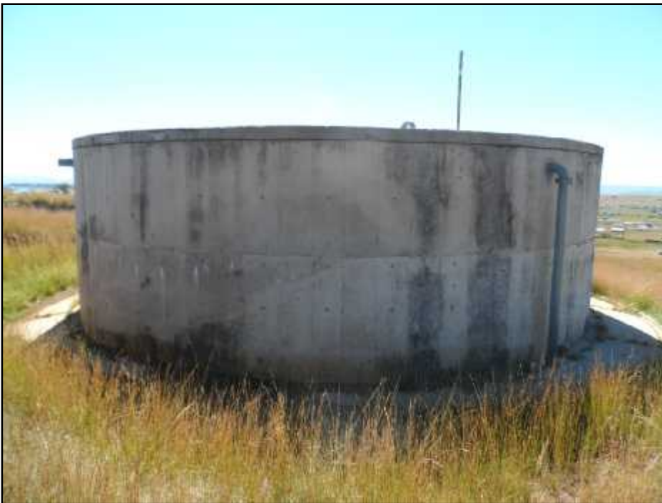
Figure 9- Reservoir located on the edges of Loskop Quarry
