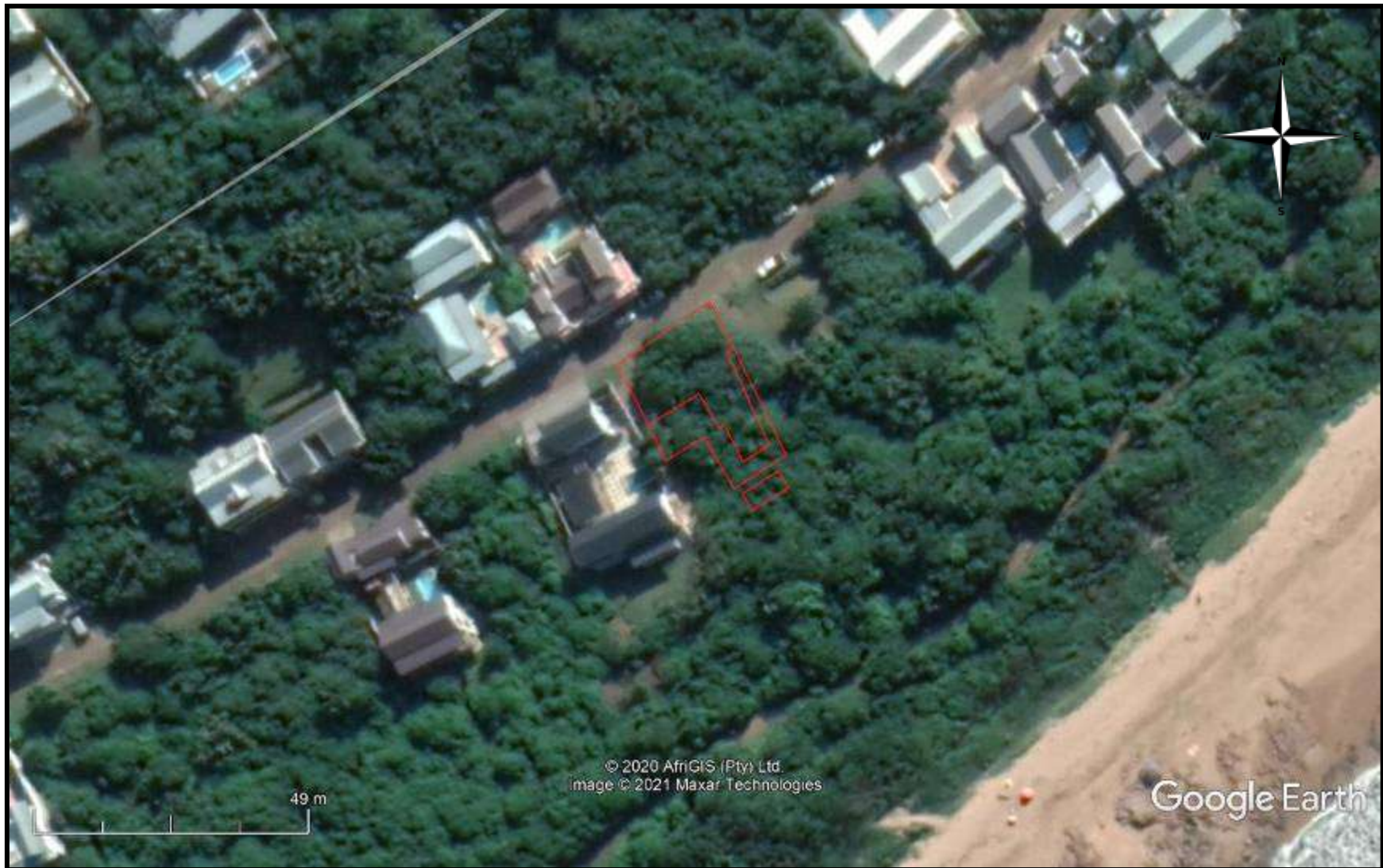
FIG. 2: AERIAL OVERVIEW OF THE PROPOSED DEVELOPMENT
