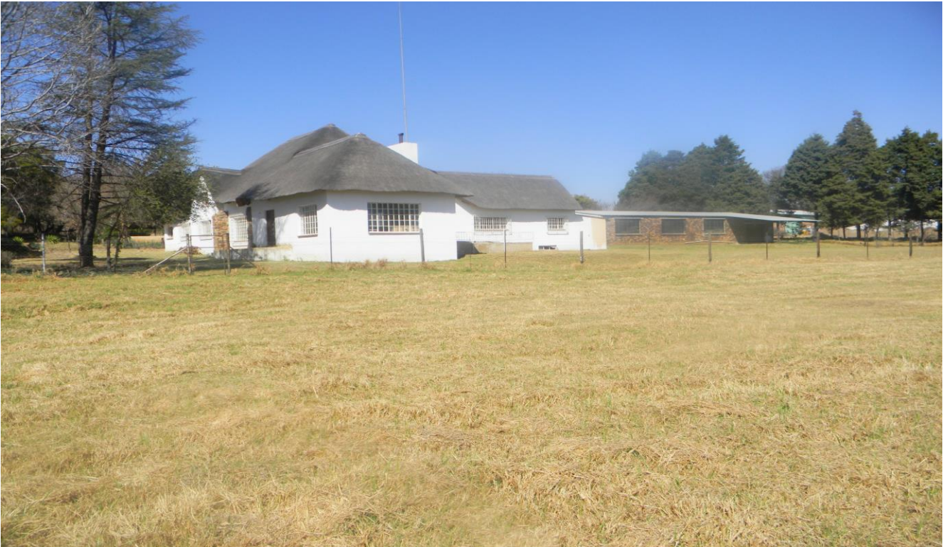
Plate 1: Photo 1: View of existing infrastructure at Magalies 2 Poultry Farm (Photograph © by Author 2017).
