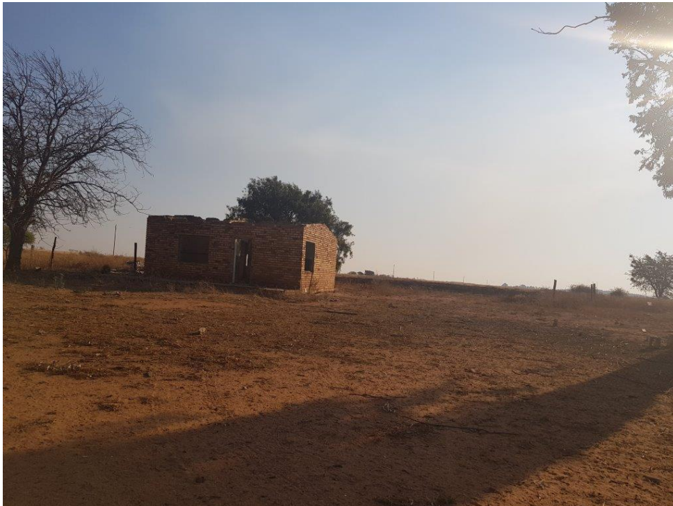
Figure 3: View of the structure currently on site.
