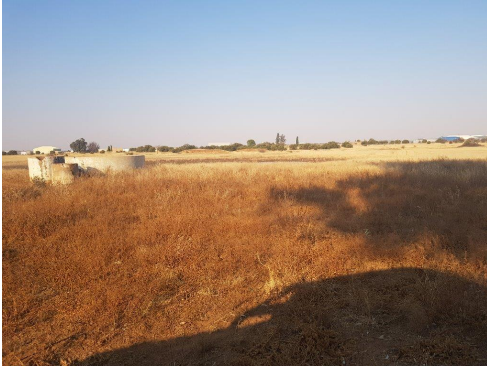
Figure 4: View of the old concrete water storage on site.
