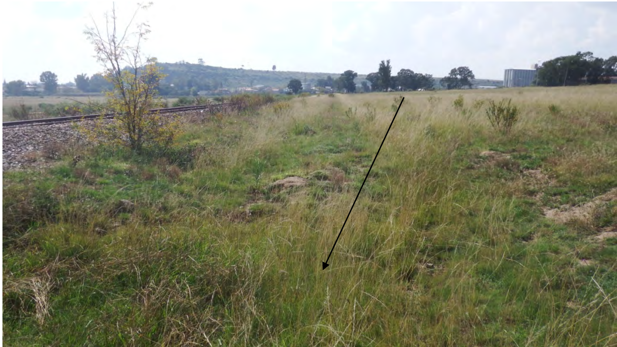
Figure 9. General view of the pipeline footprint south of the Senekal reservoir (above) and near the railway tracks (below).
