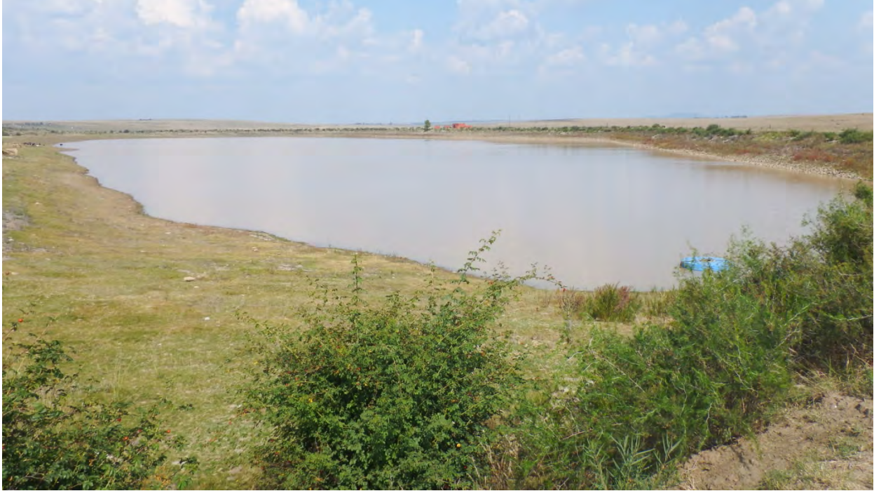
Figure 14. General view of the Matwabeng Dam, looking southeast.
