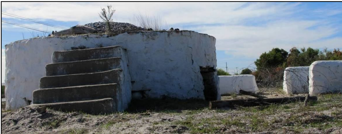
Plate 10: Lime kiln adjoining the road reserve along the Yzerfontein Road (site 007 & 008). These kilns lie immediate outside the fence line of the road reserve any may be impacted by the trench.
