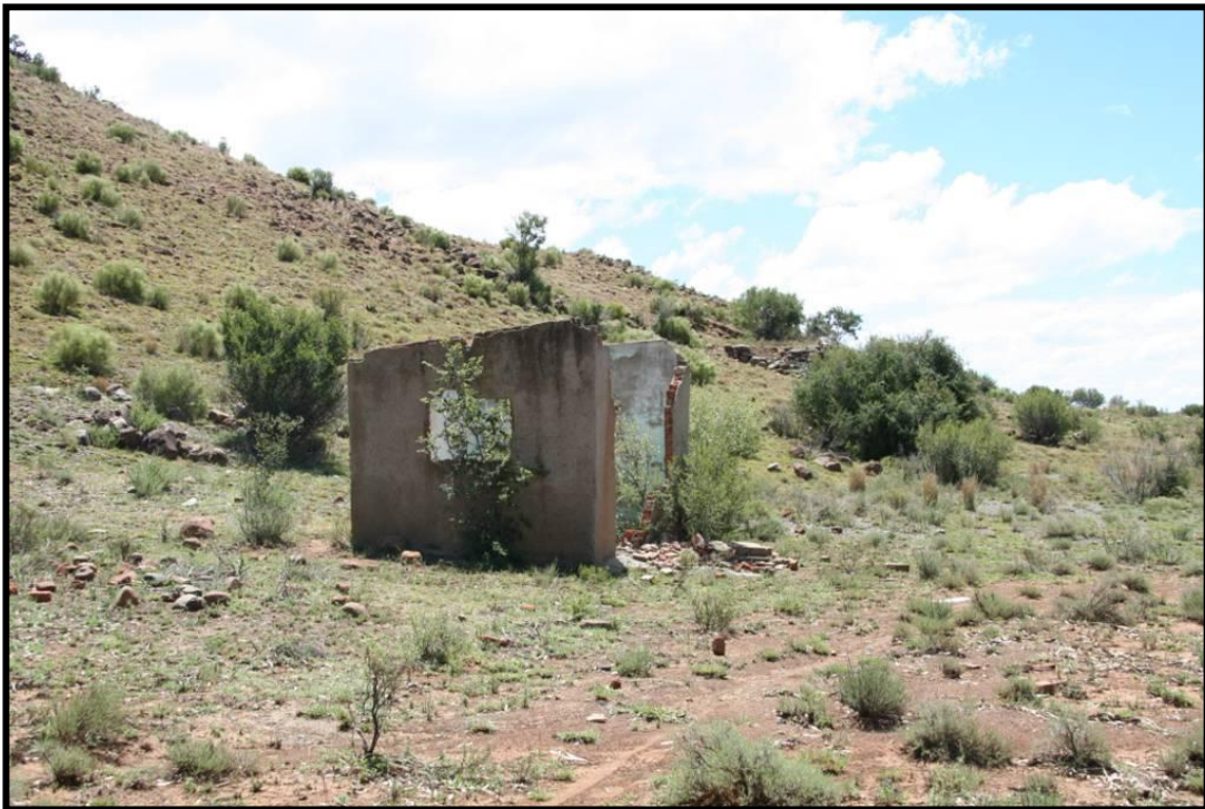
Fig. 10: Building and Platform at AN04
