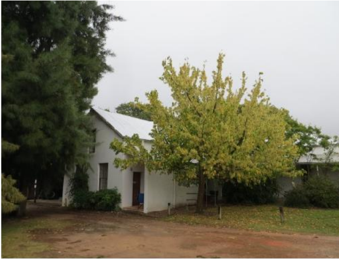
Historical farmhouse south elevation (c. 1870-80s)
