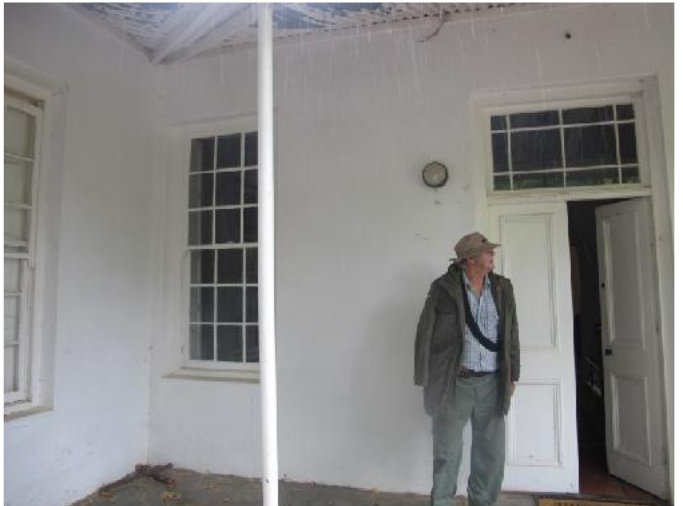
External sash window and front door detail to original structure
