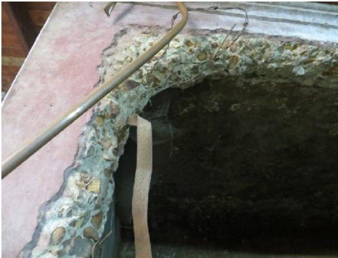
Barbed wire, stone and concrete structural detail of early wine tanks
