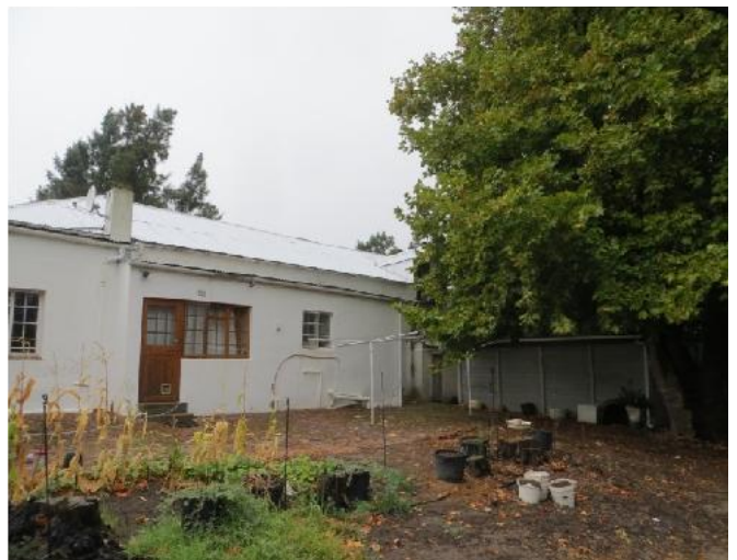
North elevation (cellar to the right)
