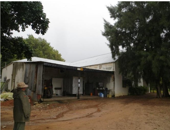
Open "afdak" extension of original "afdak" which was enclosed
