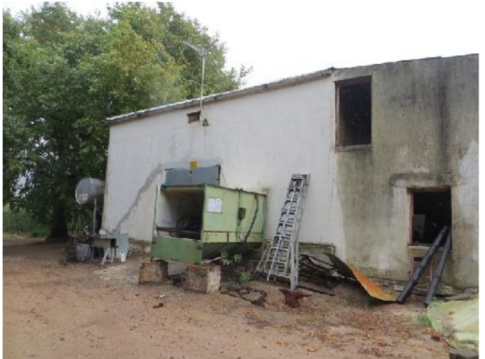
Cellar with enclosed "afdak" addition (c. pre-1938)
