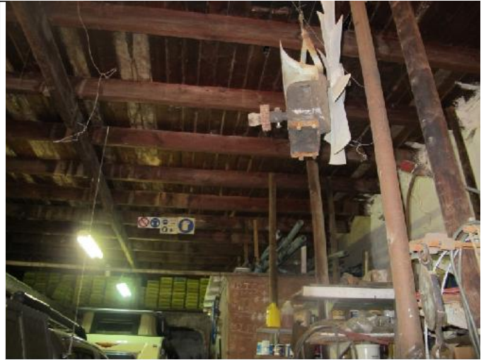
Cellar internal wooden ceiling, beams and metal pillar details
