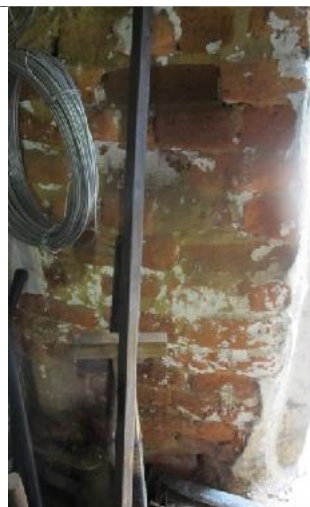
Clay brick and mud cellar walls
