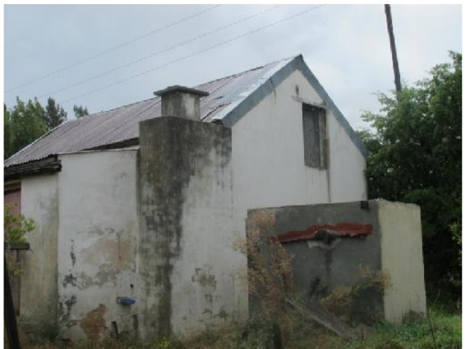
Labourer's cottage south elevation
