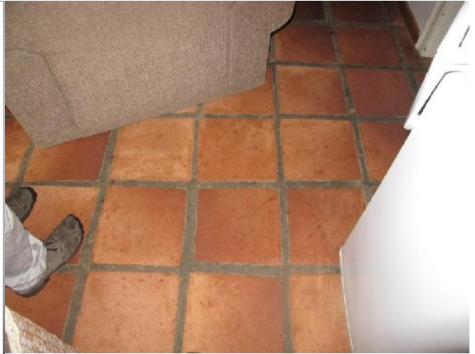
Internal terracotta floor detail
