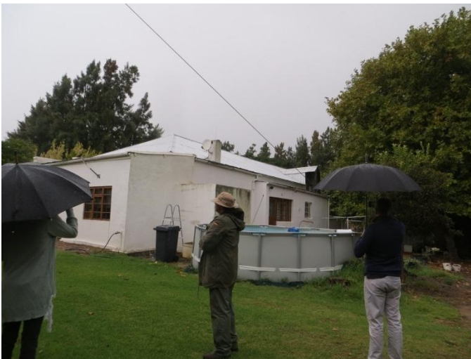
Further additions to the north elevation
