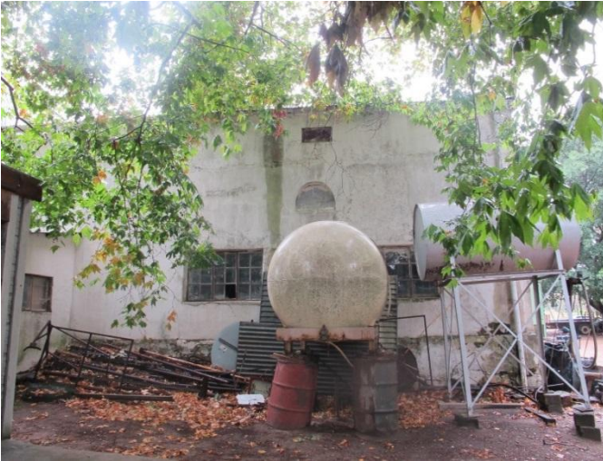
Cellar north elevation - attached to west end of the farmhouse
