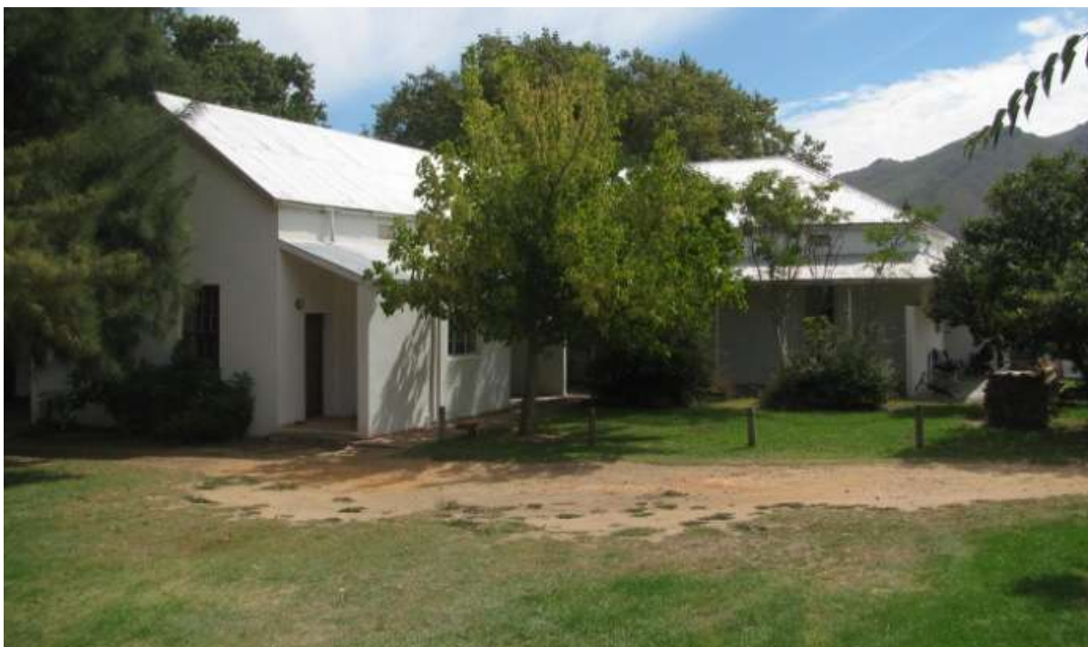
Figure 4: Historic T-shaped farmhouse, to be restored and retained
