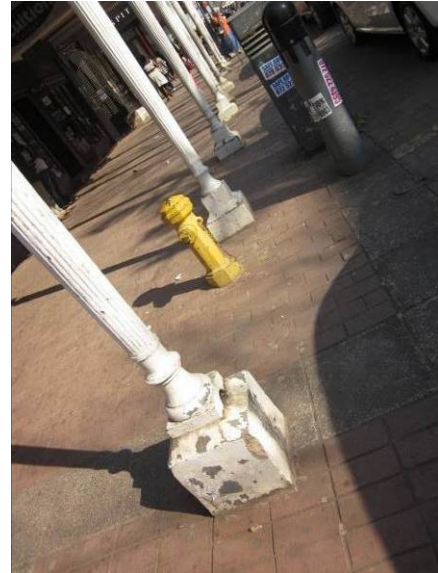
Fig 42: Supporting columns of canopies
