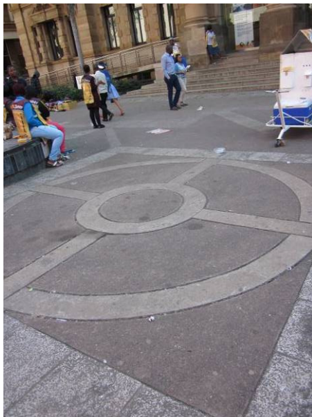
Fig 40: Current paving creating focus and space around the Gandhi Statue
