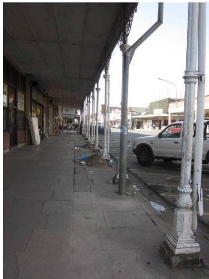
Fig 43: Canopies and posts
