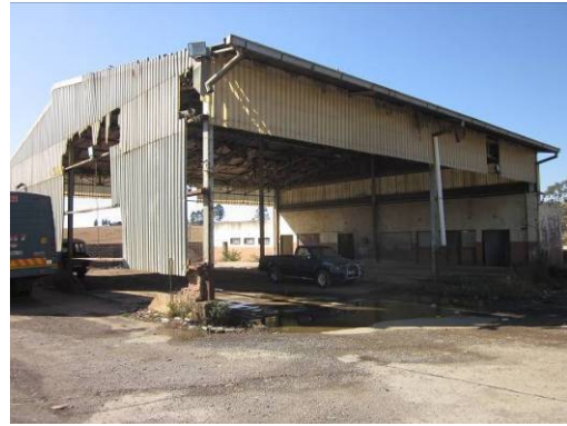
Fig 71: Bus Shed, Depot 7
