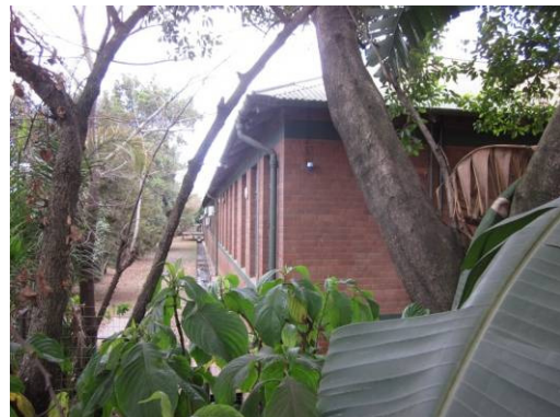
Fig 51: Proximity of old building to fence
