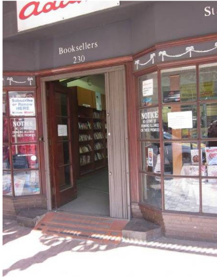
Fig 41: Old thresholds and shopfronts
