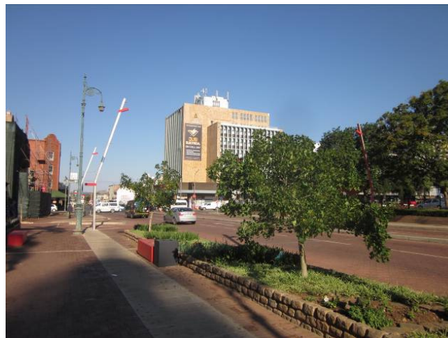
Fig 39: Showing new lighting in Chief Albert Luthuli Street
