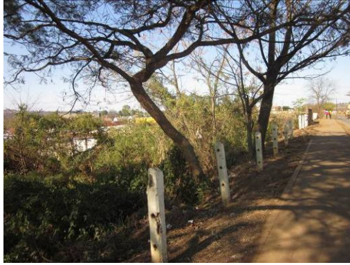
Fig 75: Post and rail fence across bridge at Depot site 8
