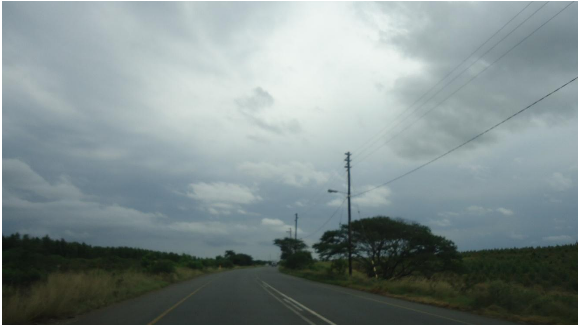
Road to be upgraded, note lack of sensitive features on either side
