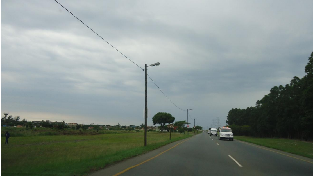
Road to be upgraded, note drainage line
