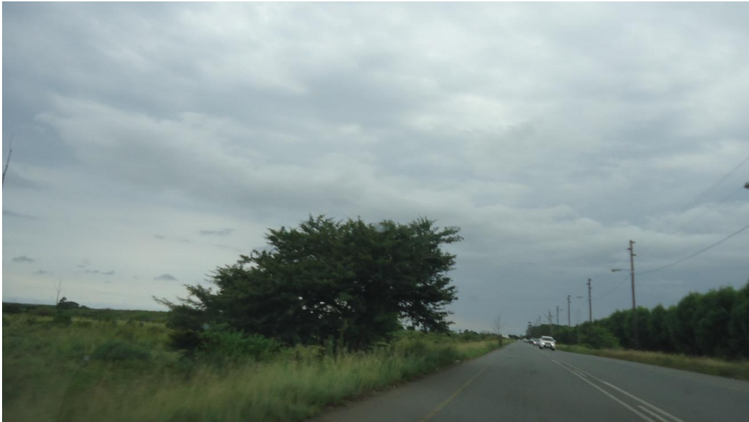
Road to be upgraded
