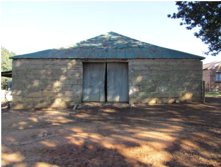
Figure 9-18: The western elevation of the sandstone barn identified at Site S.34-050 with a corrugated iron door.
