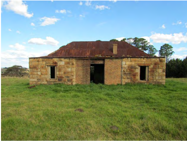
Figure 9-6: Detail of house at Site S.34-046. There as an entrance hall on the southern elevation that appears to be a new addition. The bedroom window on the left-hand side of the entrance has a metal window frame.
