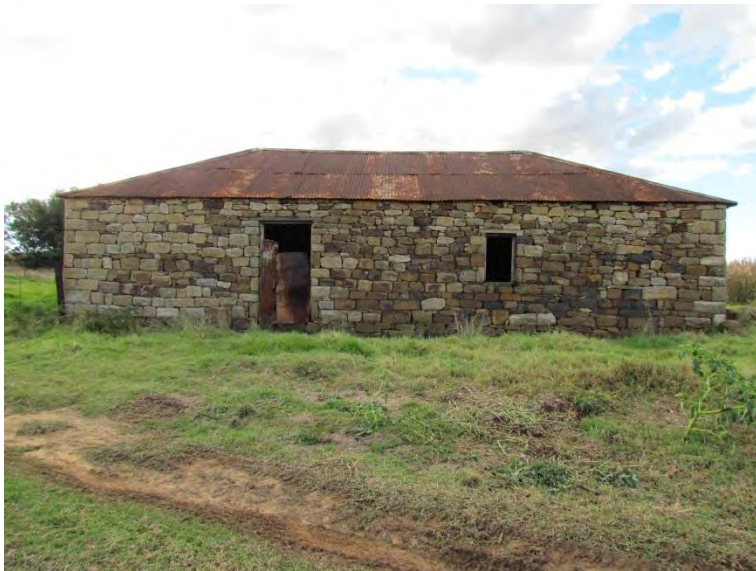
Figure 9-11: The northern elevation of the barn has one door and one window.
