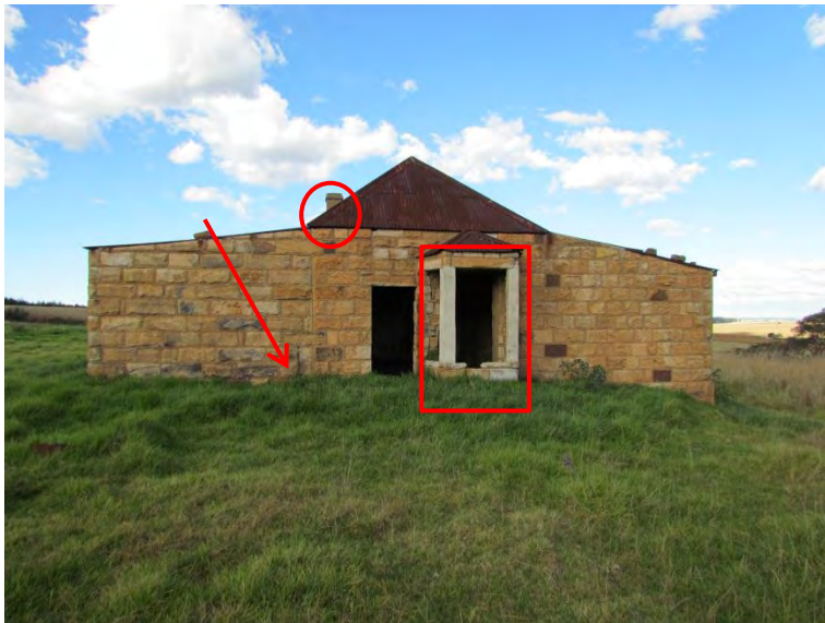
Figure 9-2: Detail of house at Site S.34-046. An entrance and a bay window (red square) are situated along the eastern elevation. This entrance leads into the living room which has a fireplace, indicated by the chimney (red circle). There is also a pipe on the exterior wall (red arrow).
