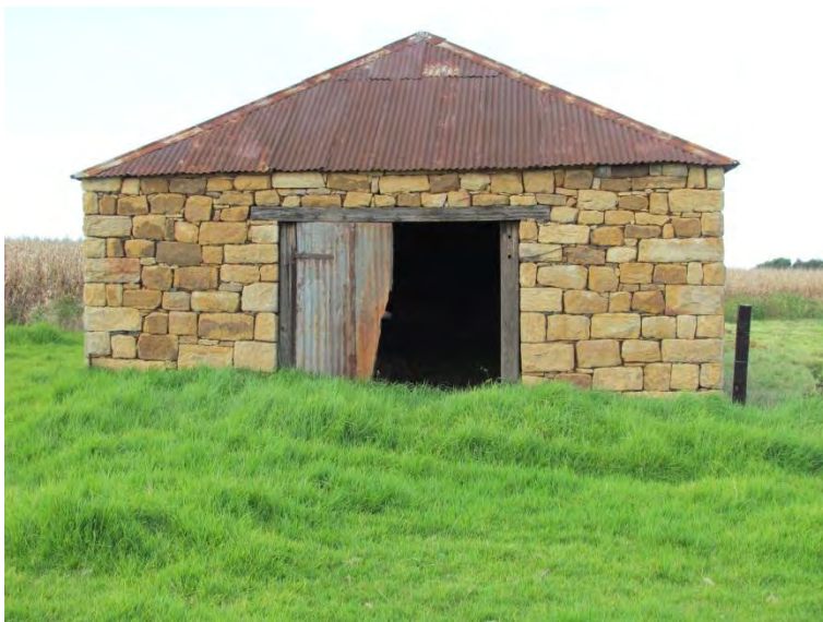
Figure 9-9: The sandstone barn with a corrugated iron door and a wooden door frame on the eastern elevation at Site S.34-046.
