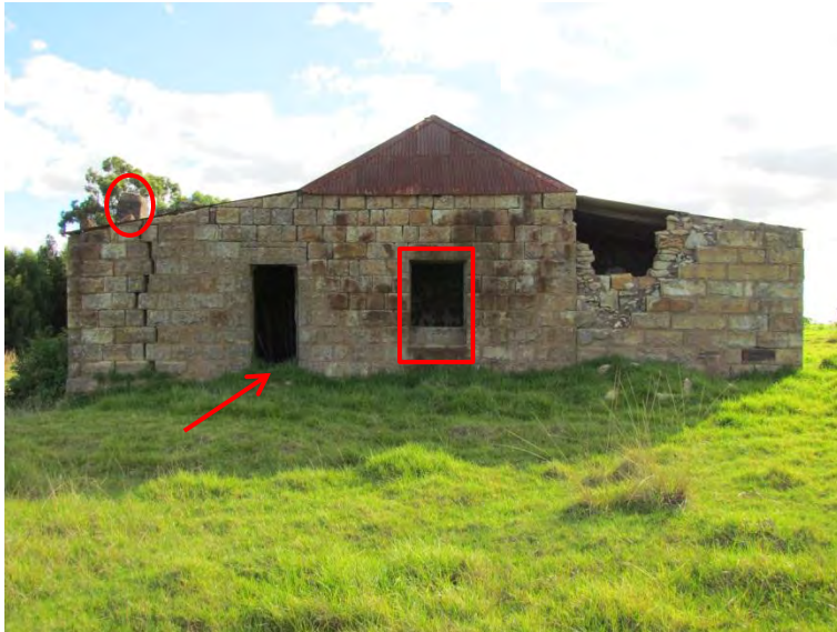
Figure 9-4: Detail of house Site S.34-046. The western elevation has steps leading in a kitchen (red arrow). There is a bedroom on the right-hand side and far right-hand side (red squares). The kitchen has a fireplace, indicated by the chimney (red circle).
