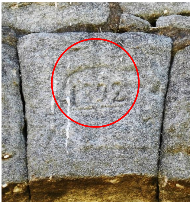
Figure 8-7: Detail of keystone of S.34-001 dating the building to 1892.
