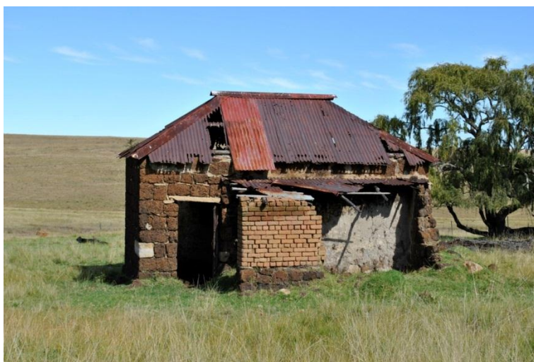
Figure 8-5: S.34-002 – Original farmhouse. Note later addition as indicated by sunbaked bricks.
