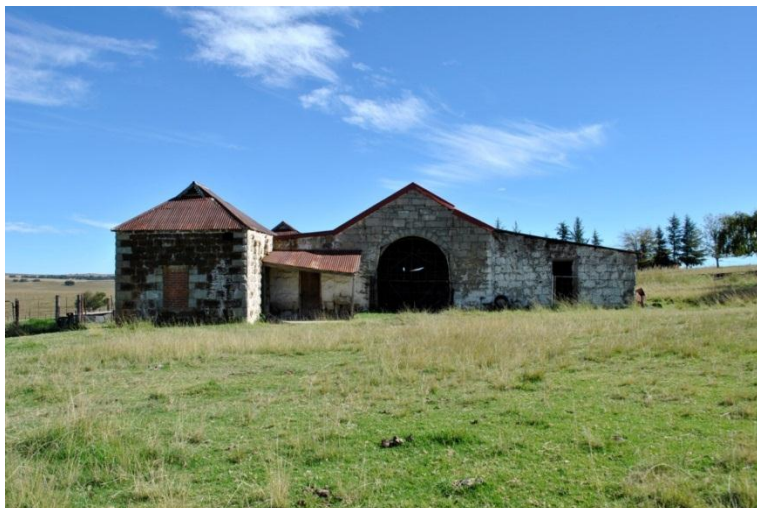
Figure 8-6: S.34-001 – Old milk-shed dated to 1892. South facing section.
