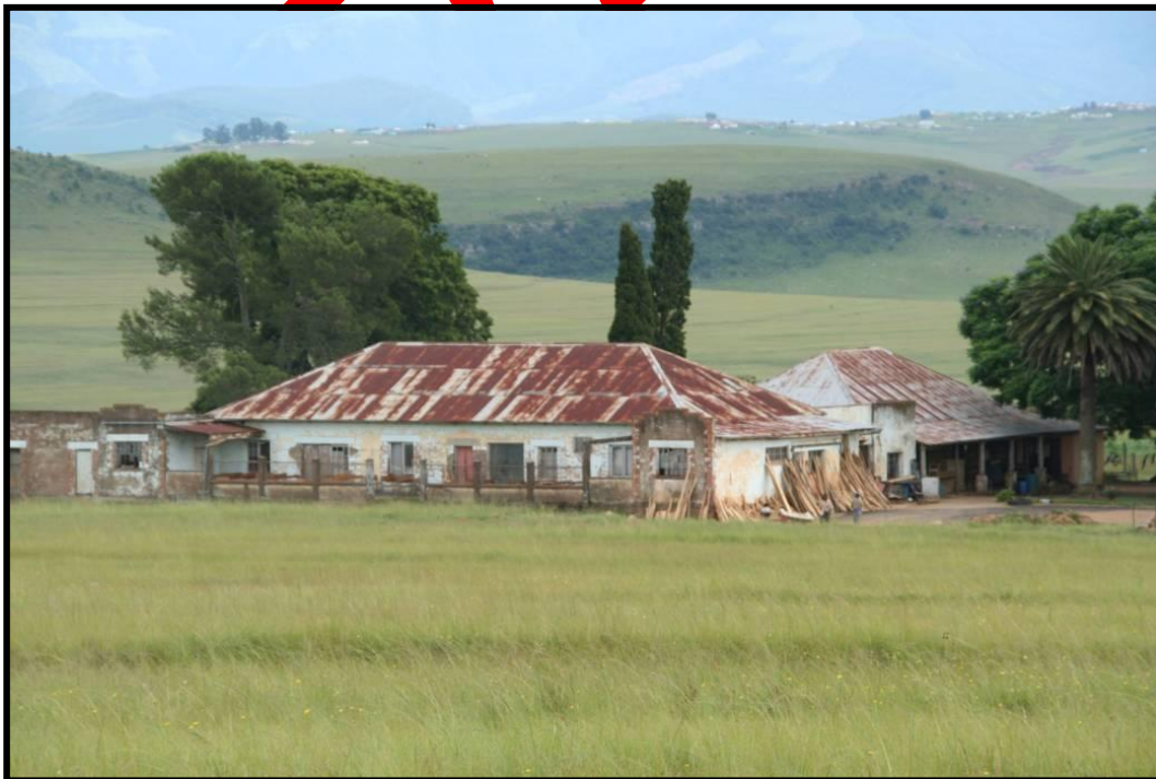
Fig. 14: Buildings At UMT08
