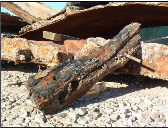
Figure 3: Possible wooden shipwreck structure
