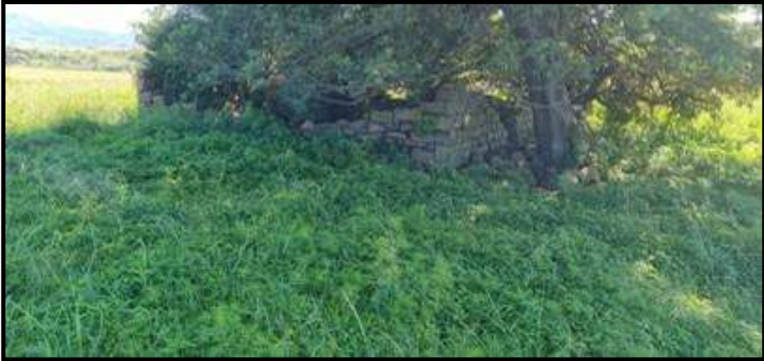
FIG. 21: BUILT STRUCTURES AT MUL02
