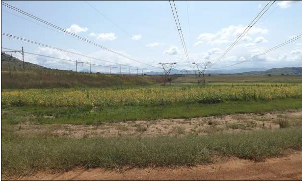
Figure 5: Image showing the railway line embankment, Eskom electricity powerlines and the low-rouned hills to the north.
