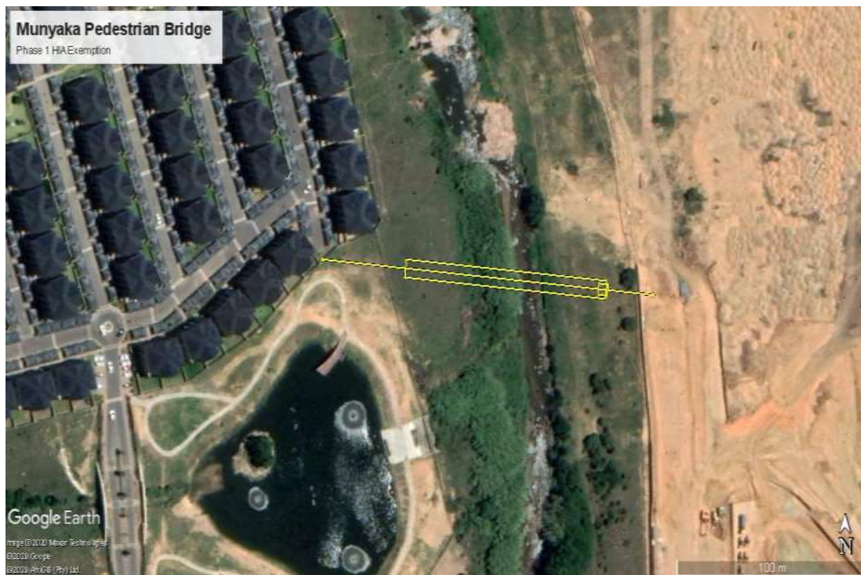
Figure 2: Closer view of location of proposed Pedestrian Bridge (Google Earth 2020 – Estimated footprint of bridge provided by Bokamoso Landscape Architects & Environmental Consultants CC).
