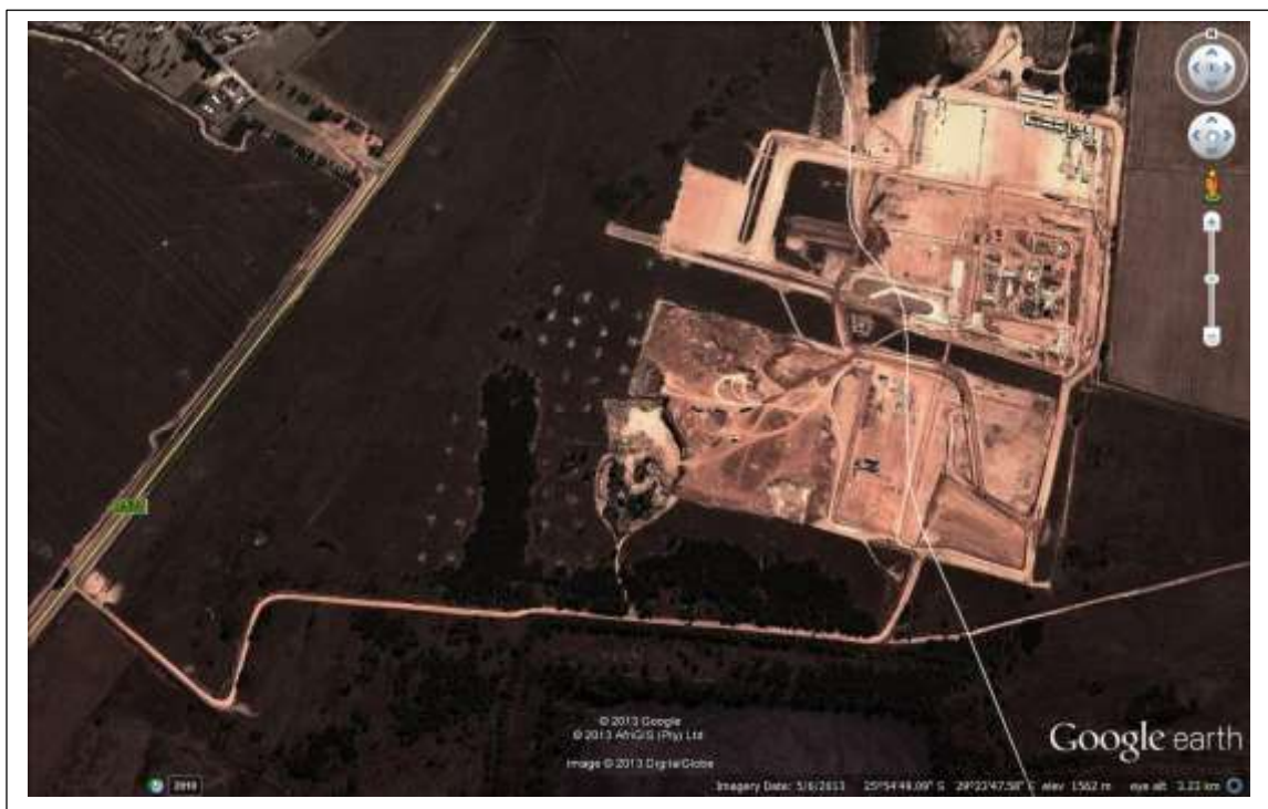
Figure 3- The clean water pipeline commences within the MWTP which is currently under construction. This part of the project area has totally been altered by developmental activities (above).
