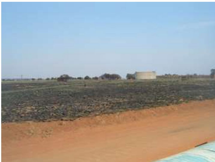
Figures 7, 8 & 9- The penultimate stretch of the clean water pipeline runs across abandoned agricultural fields (top and centre) whilst the last stretch crosses a conveyor belt before ending at a reservoir (below).
