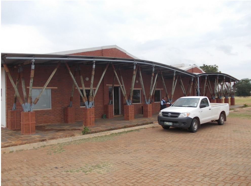
Fig 2. View of existing sisal processing factory
