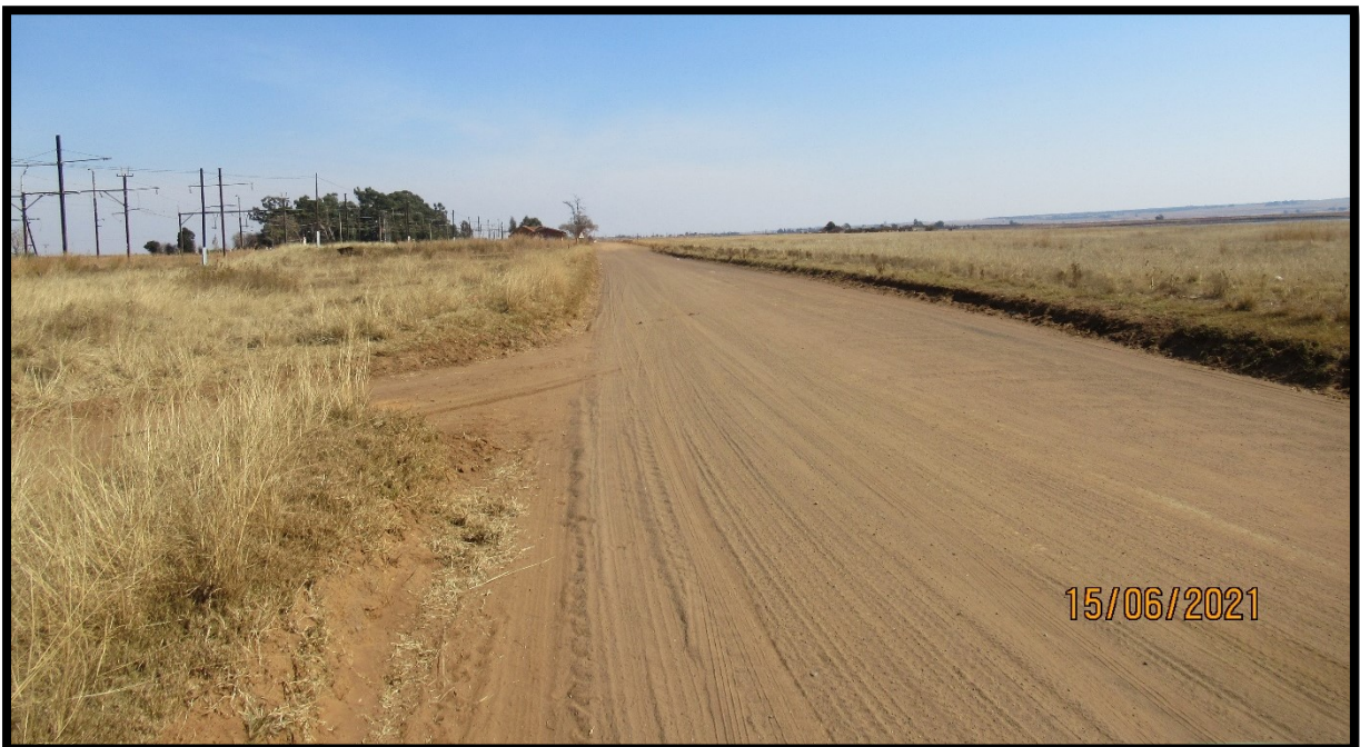
Figure 7: View of road towards railway line.
