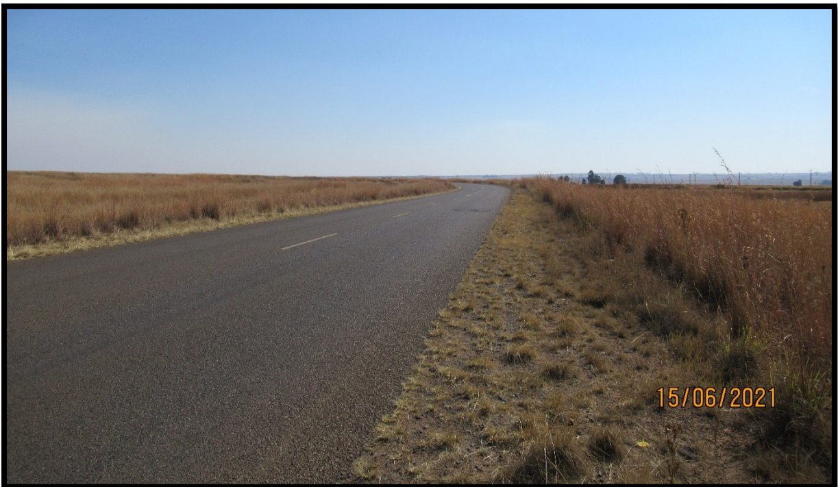
Figure 11: View of R104 Road where the new access road will join.
