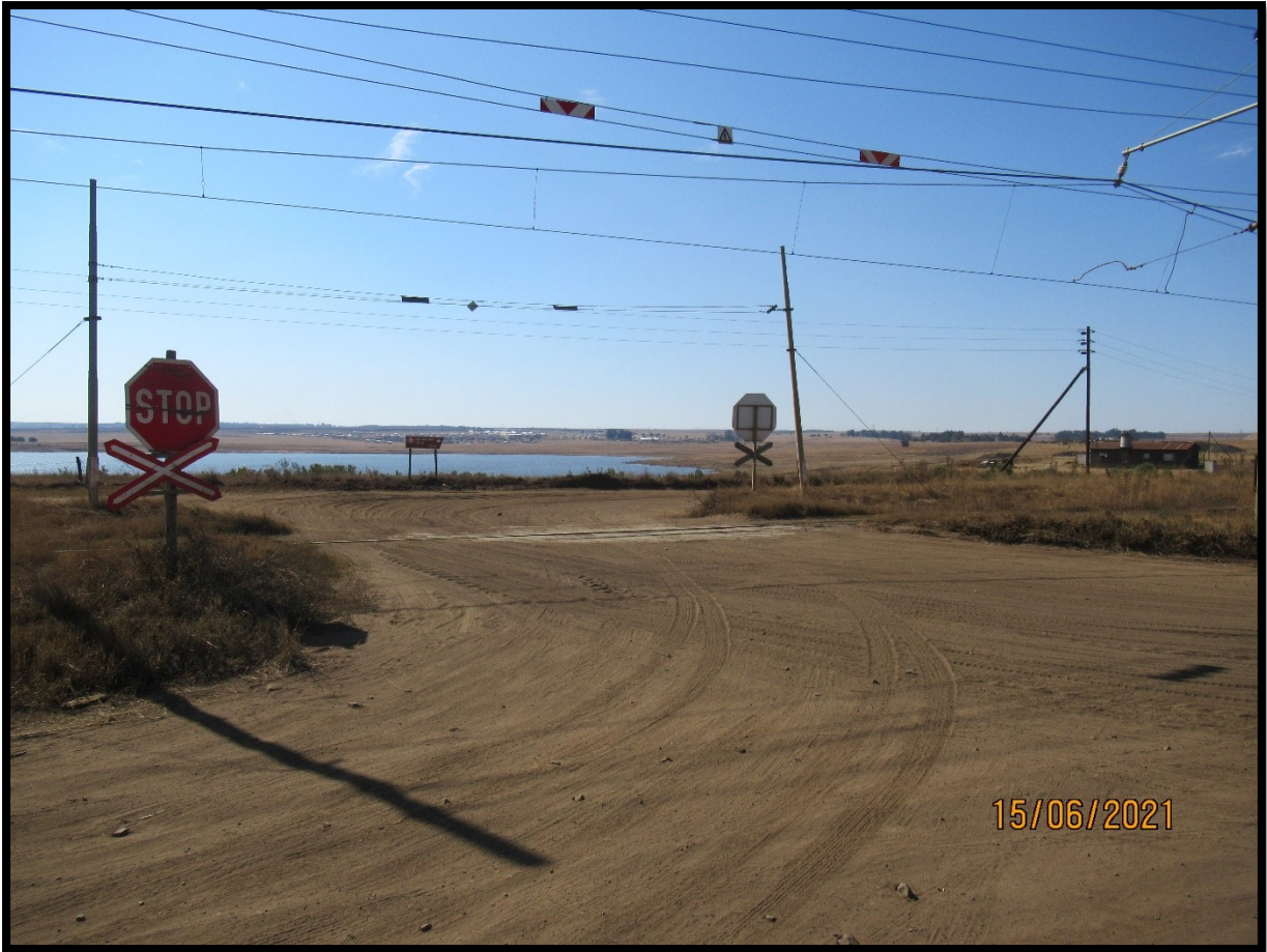
Figure 8: View of railway crossing.
