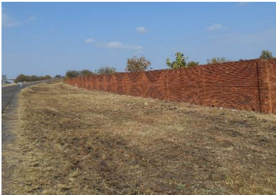
Figure 3: Road reserve of N1
