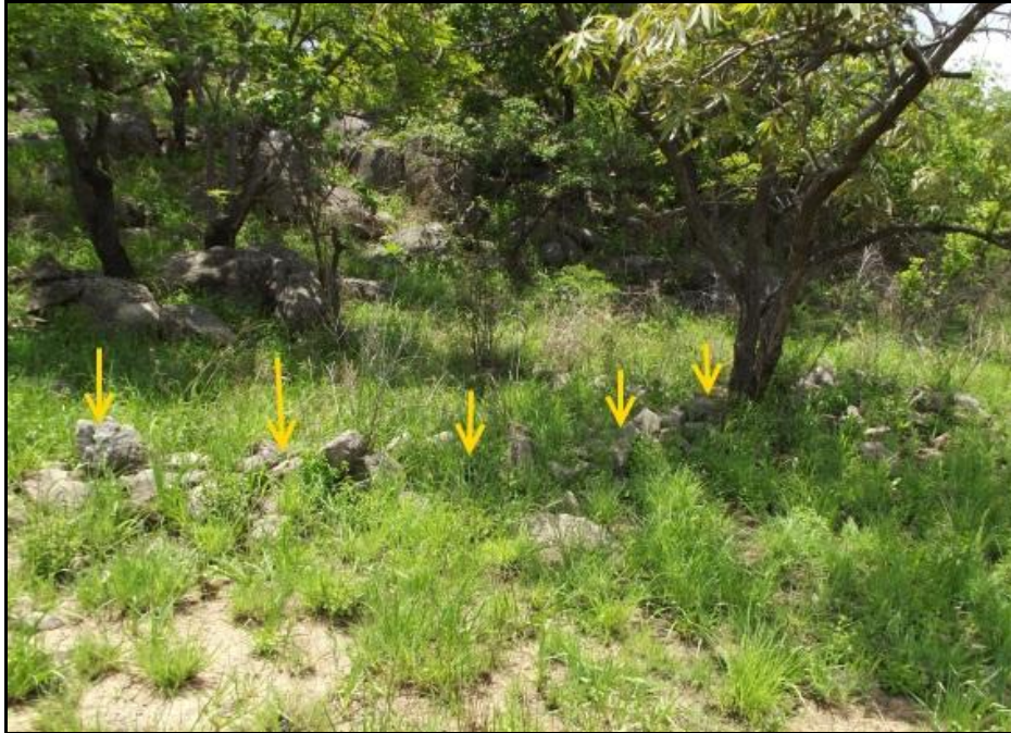
Fig. 21. Site MAN 15. Linear stone walling located a few metres north of site MAN 14.
