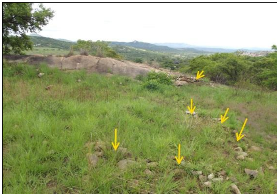
Fig. 12. Site MAN 9. Ruins, arrows indicate where the foundations of the building were. North of site MAN 8.
