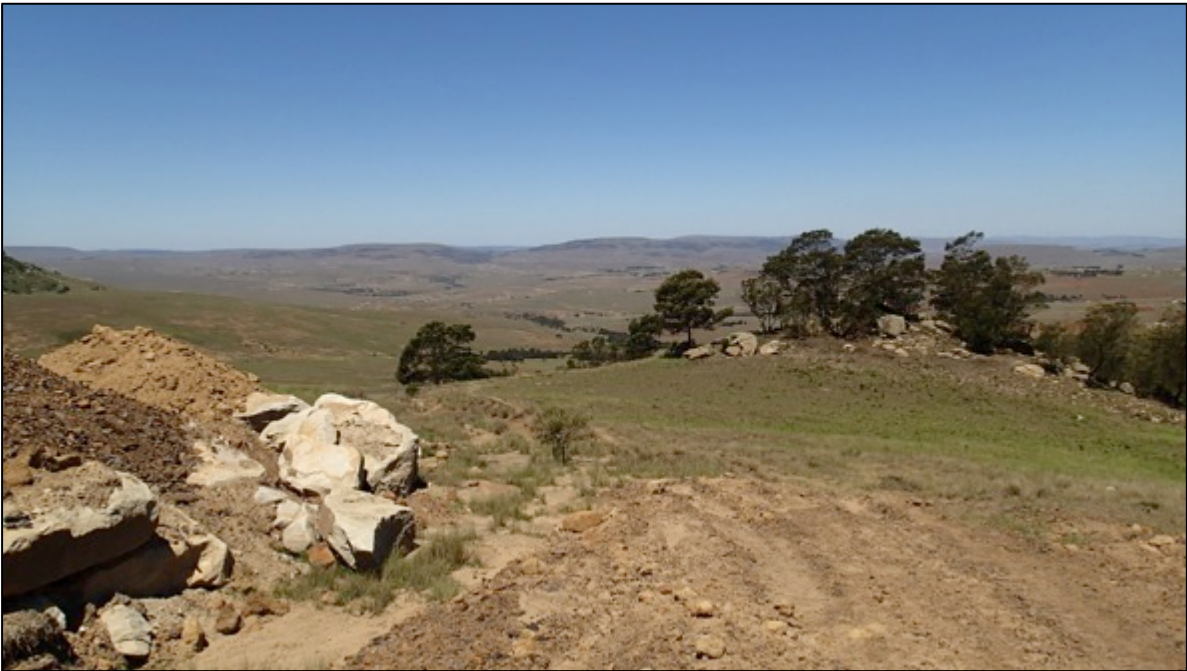
Figure 6. Magogo road upgrade
