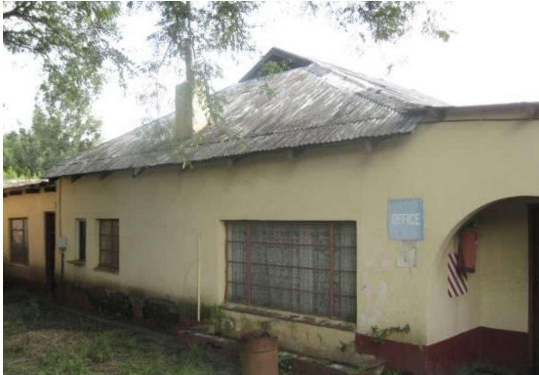
Figure 17. Nineteen sixties farmhouse, previously used as the mine office.
