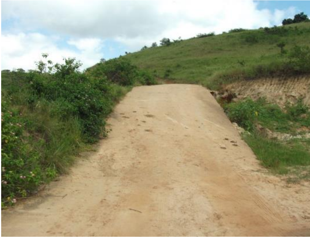
Figure 4: View of bridge and associated erosion
