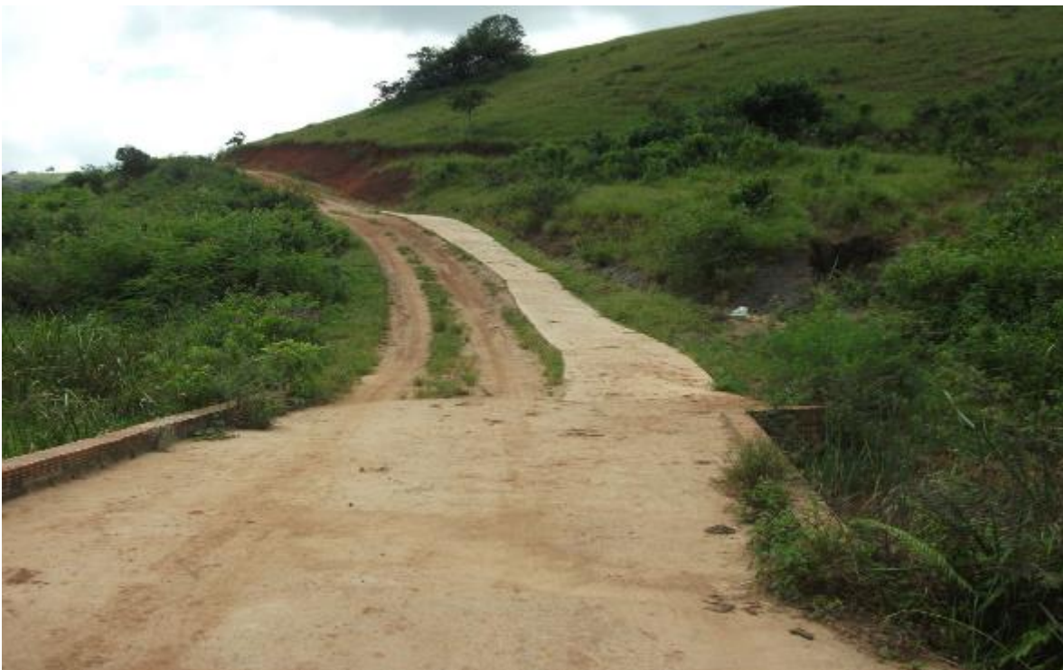
Figure 3: View of existing bridge
