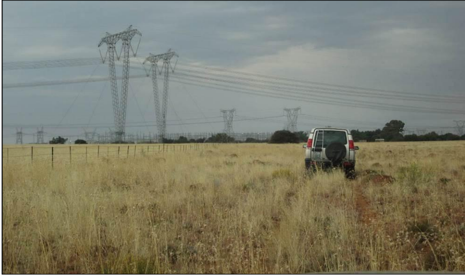
Figure 20: View southwards towards the farm werf (in the trees) on Walvischkuil. The Beta substation is visible in the background on another farm.
