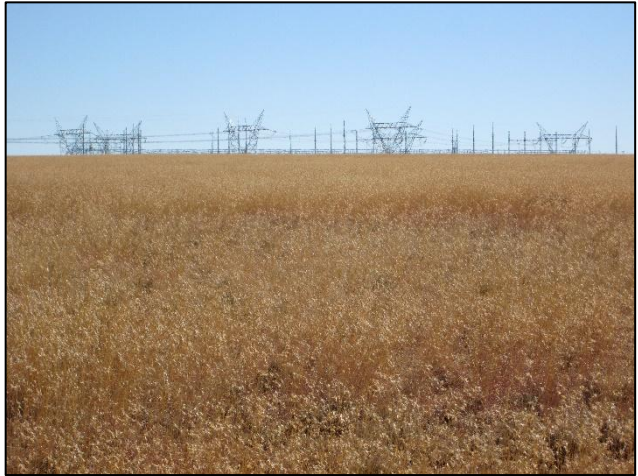
Figure 8: View over the southern part of Kentani towards the Perseus Substation to the north.
