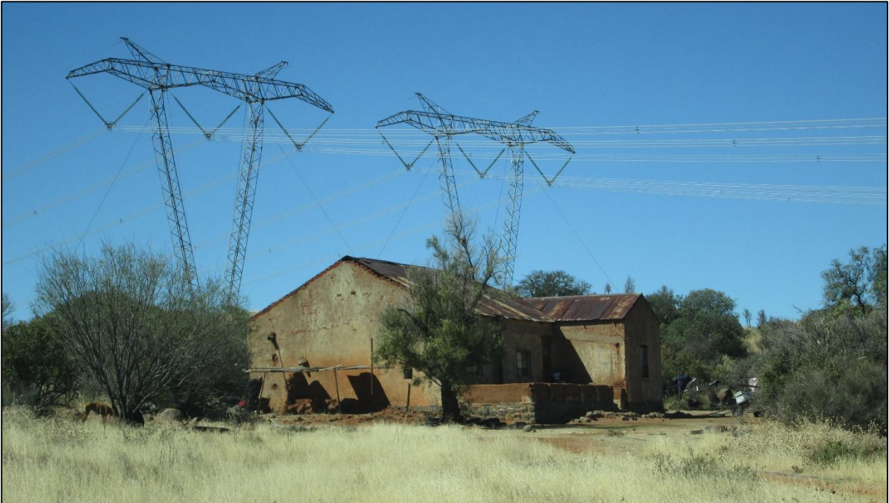
Figure 59: The northern end of a historical house on Doornrandjes (point 099).
