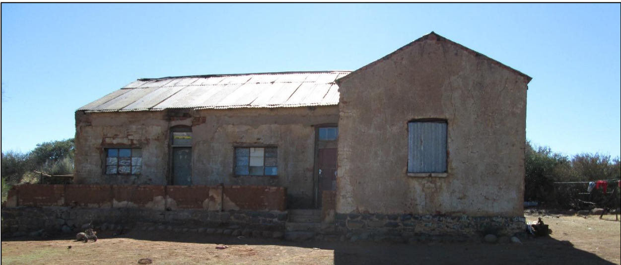
Figure 58: The west-facing façade of a historical house on Doornrandjes (point 099).
