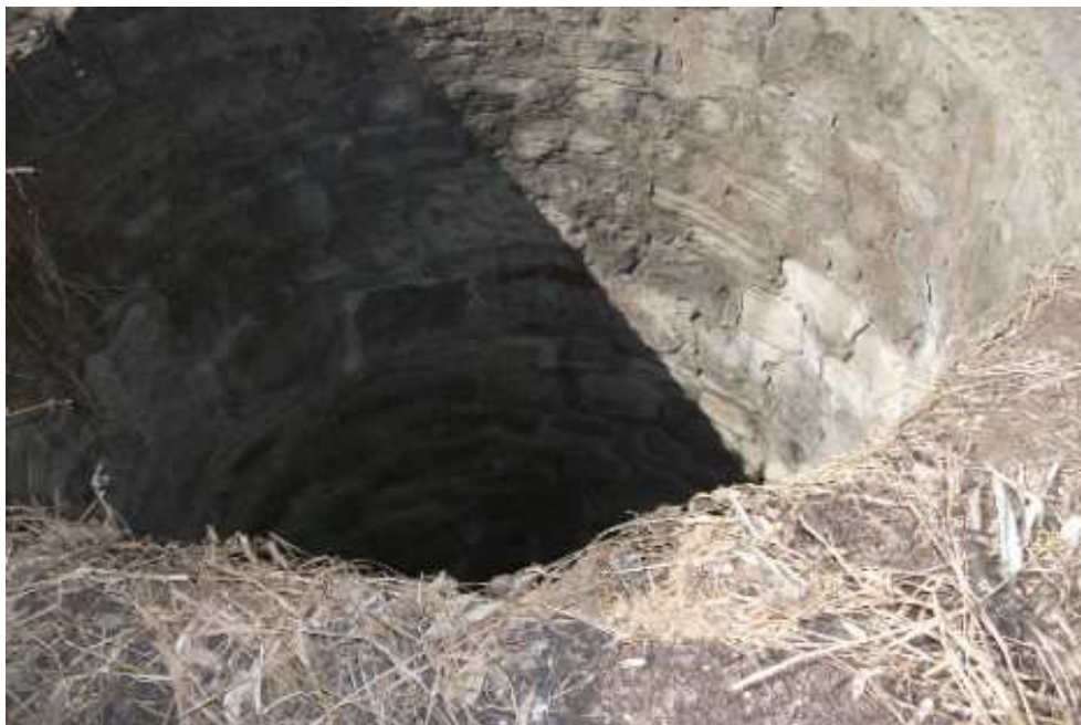
Figure 7: Inside of stone structure
