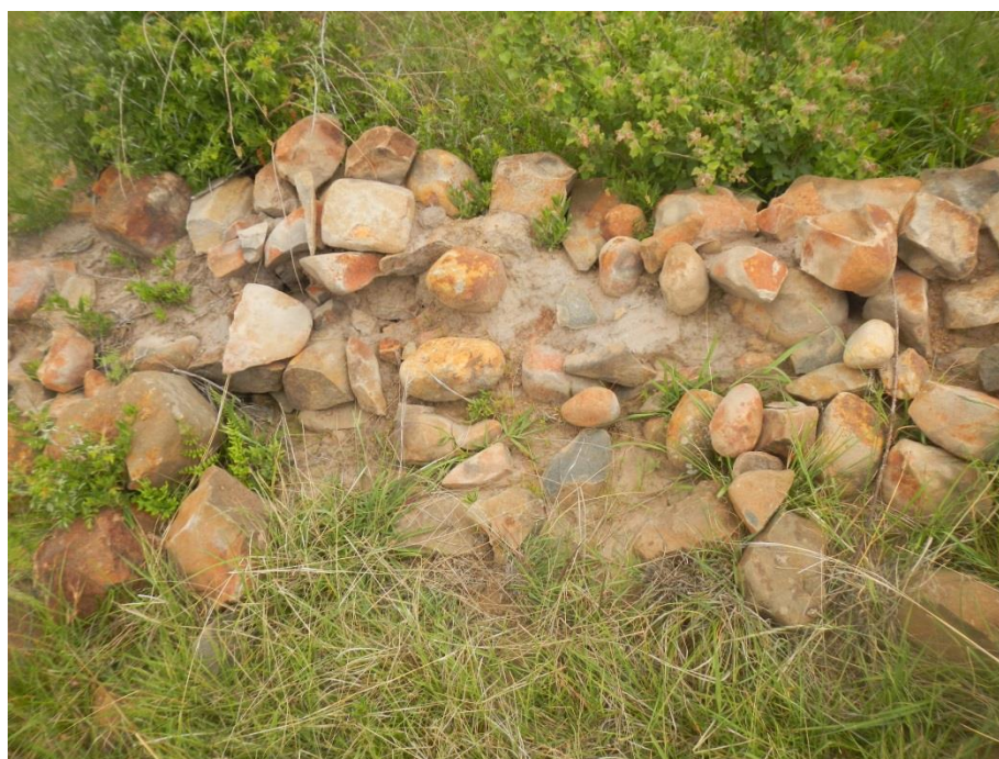
Figure 4: View of part of the stone walls joined with mortar
