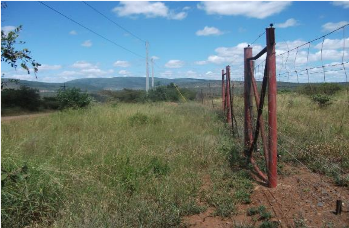
Figure 12: Pipeline route between road and game fence
