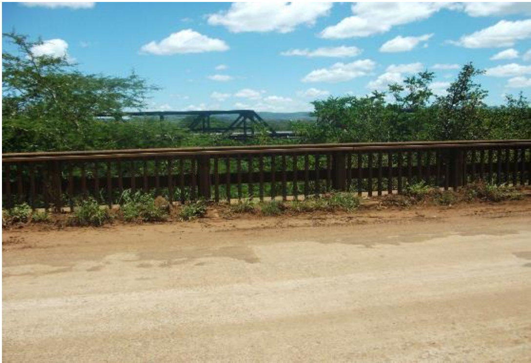
Figure 19: Road bridge with rail bridge in background
