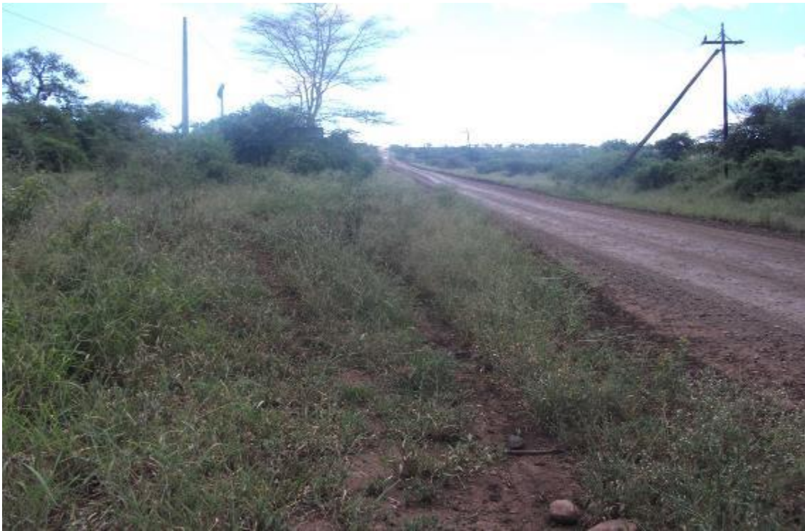
Figure 11: Pipeline route near watercourse
