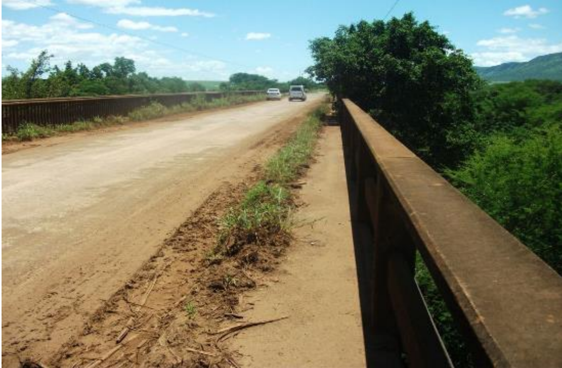
Figure 18: Road bridge over Mkuze River
