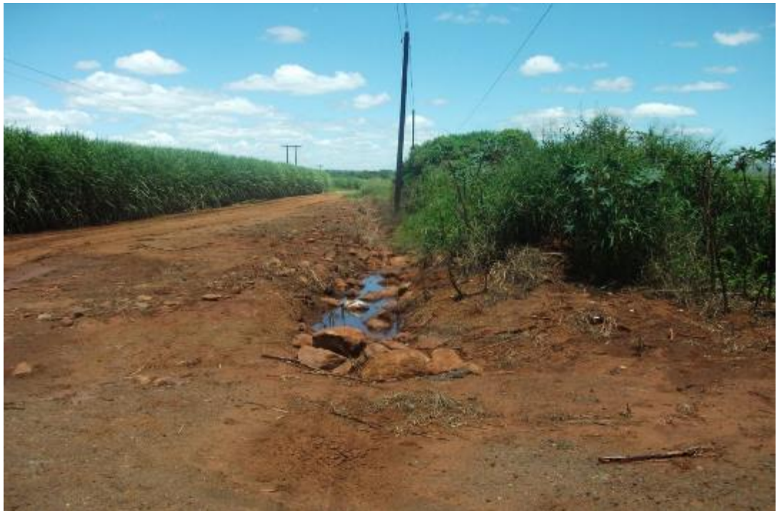
Figure 20: Pipeline route adjacent to road
