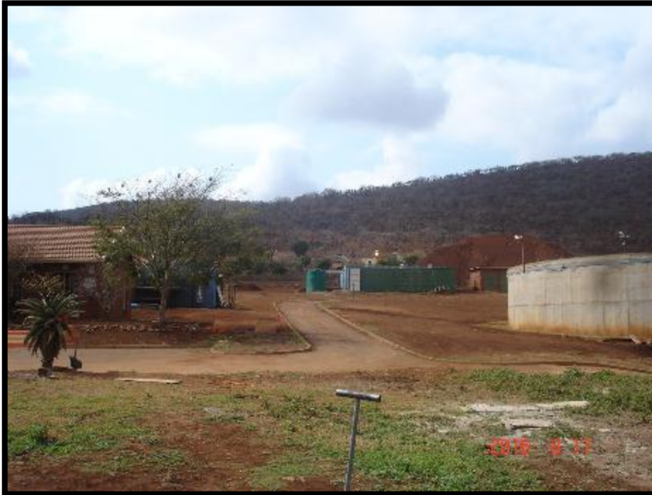
Figure 7. The Mandlakazi Water Purification Works.
