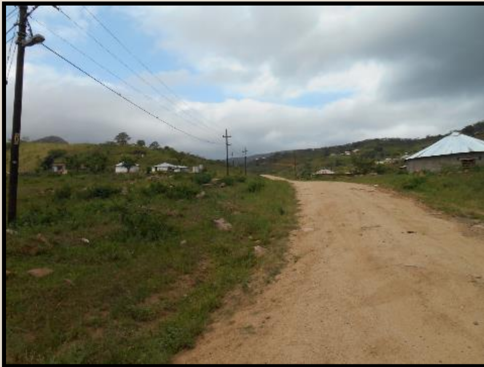
Plate 4. Preferred Site of Pump Station 1.
