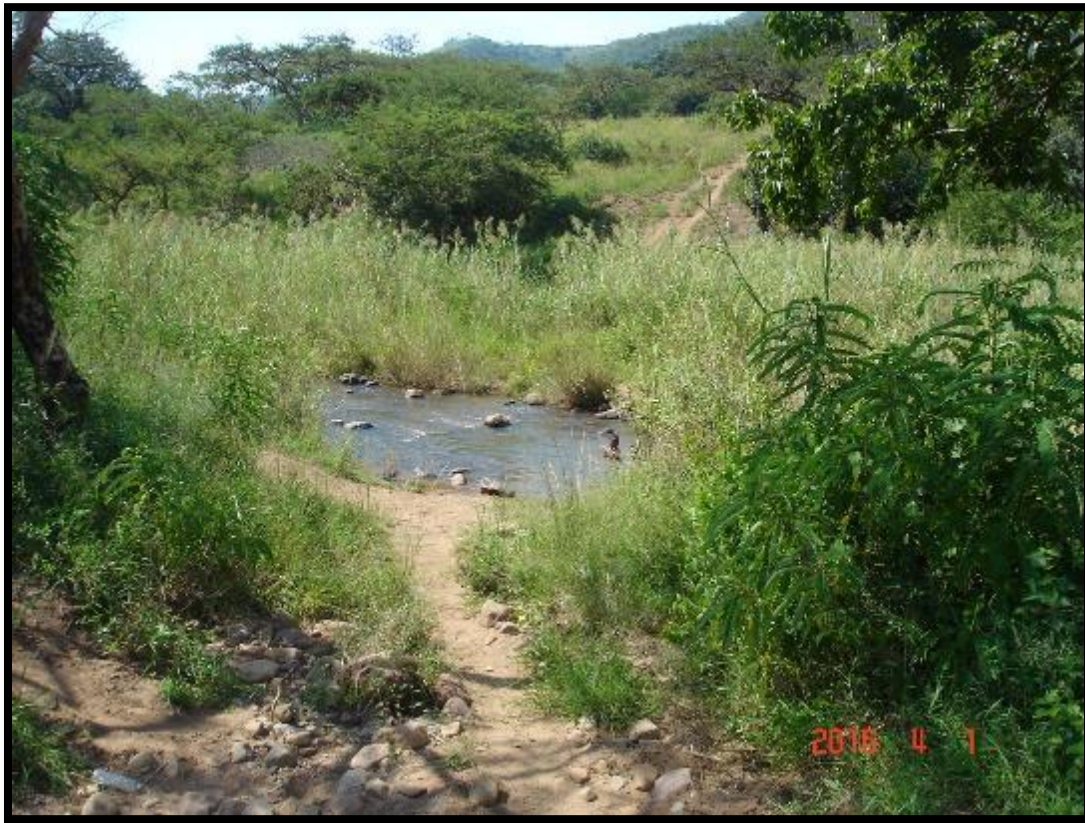
Plate 1. Site of the proposed Maphumulo Causeway (photograph by S Whitaker).
