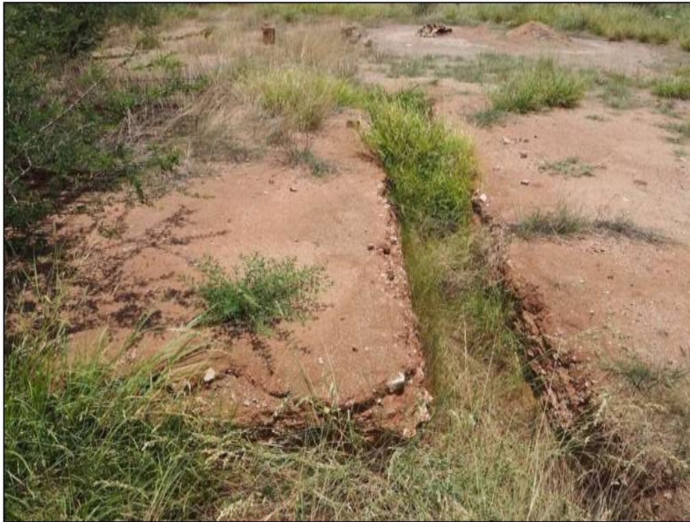
Figure 23. Finished foundation excavations
