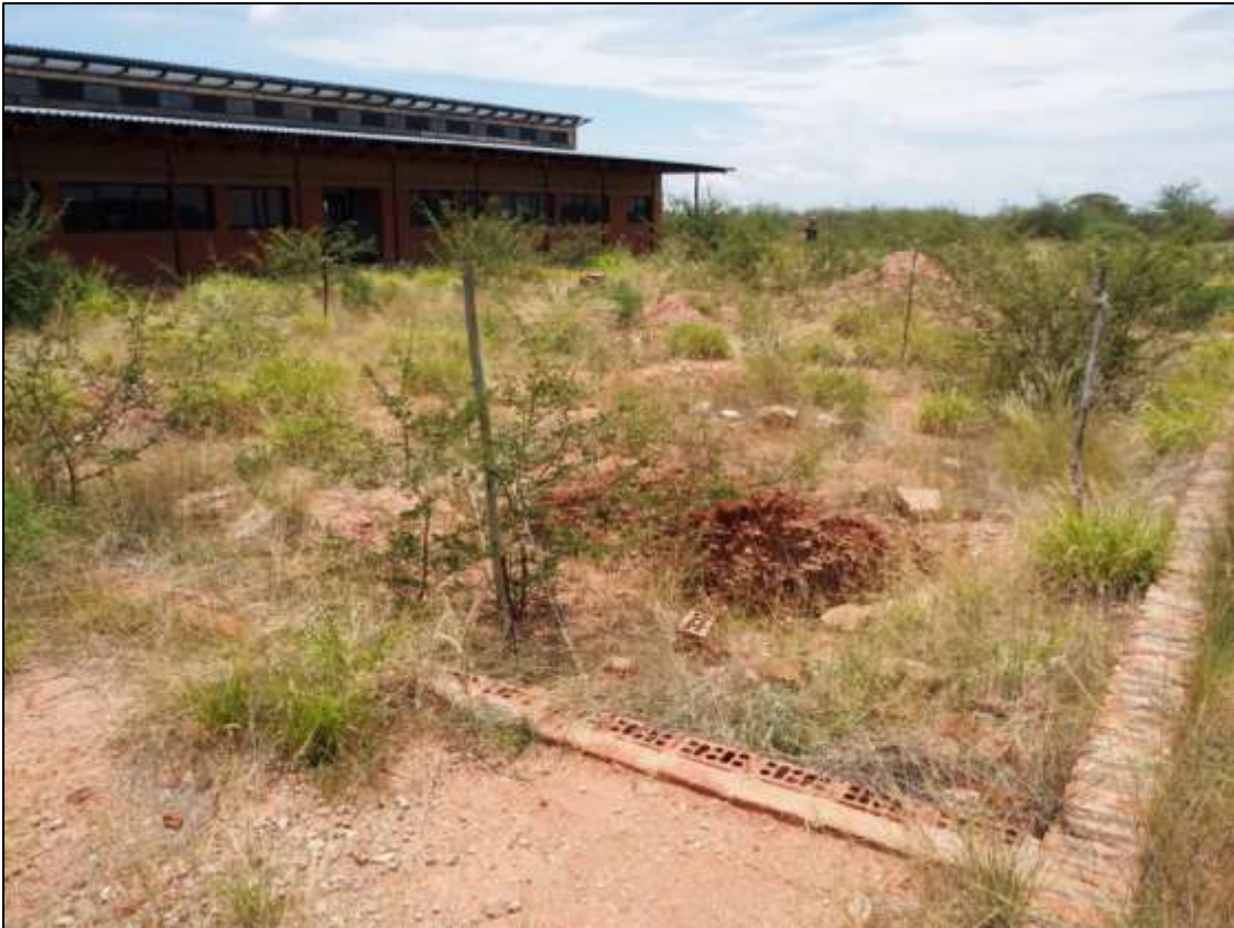
Figure 21. Foundations of structures still to be finished
