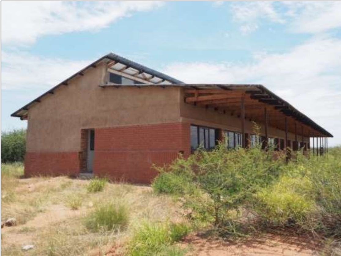
Figure 20. Largely finished Office Complex structures
