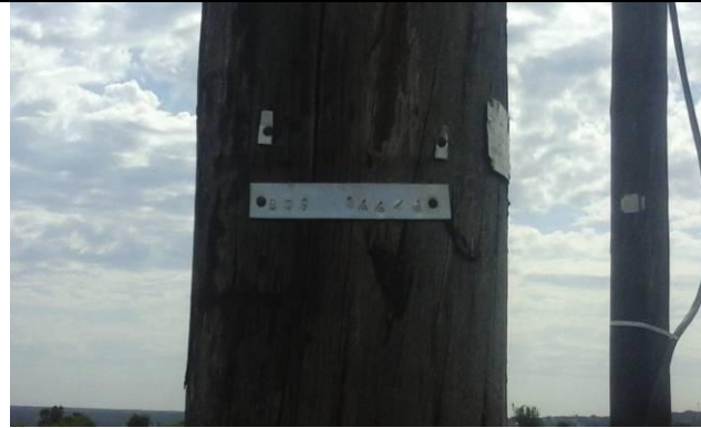
Fig 1: View of pole DMG144/1
