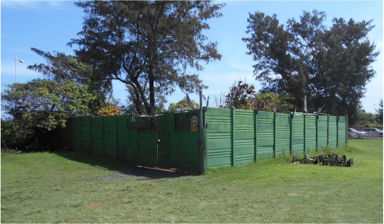
Figure 7: Pre-cast walled area
