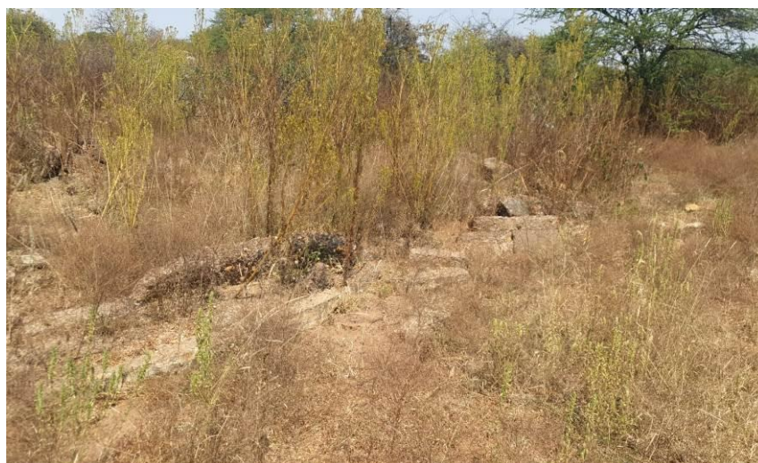
Fig 11. Remnants of a residential building (2)
