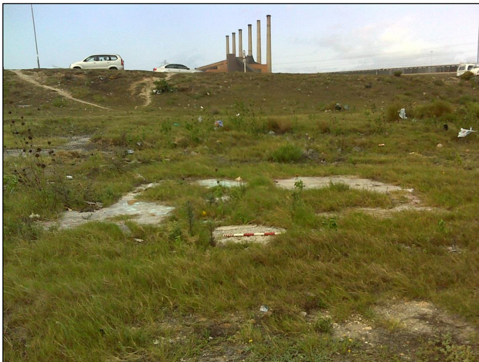
Figure 8. Close-up view of one of the remaining built environment foundations occurring within the proposed development site.
