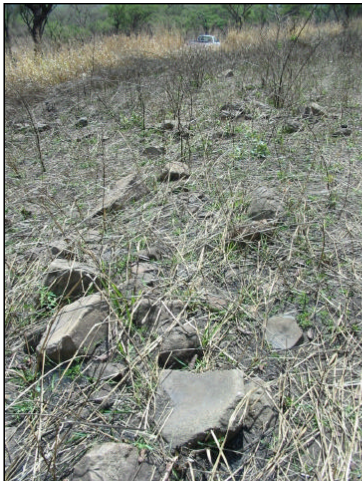
• Figure 15: Dry stone walling
