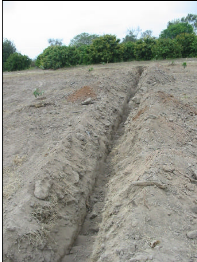
• Figure 36: Trench through site
