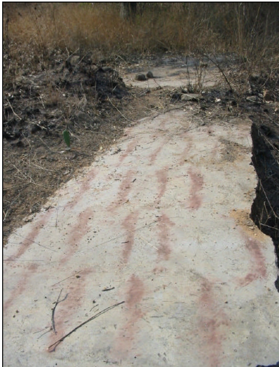
• Figure 32: Cement Floor
