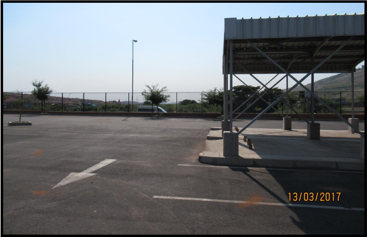
Figure 6: Different view showing empty lot to the east and taxi rank in view to the right.
