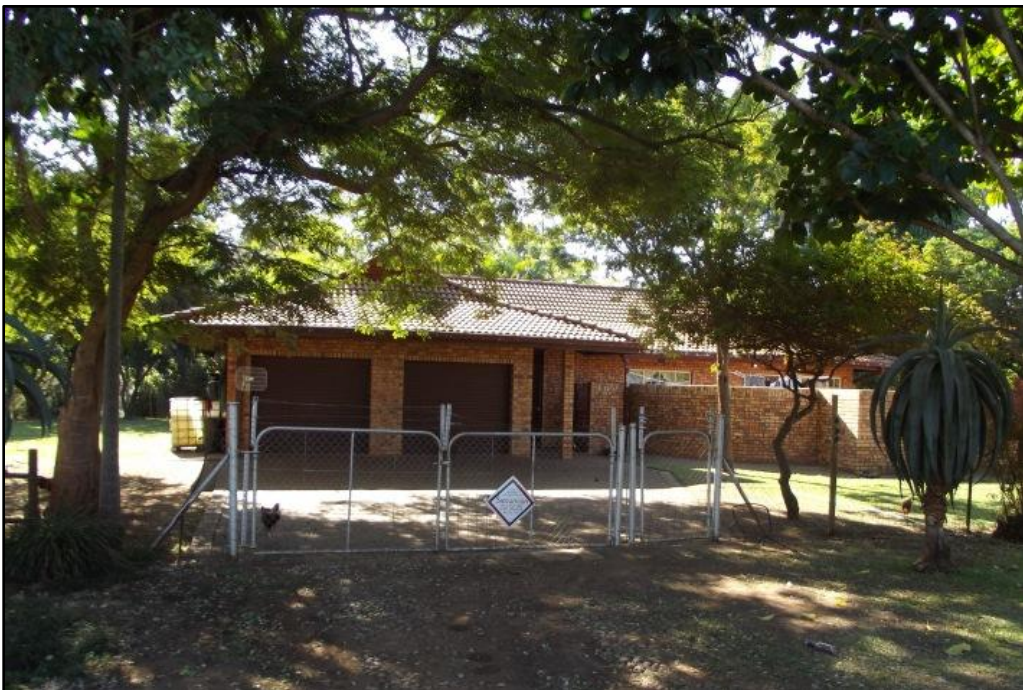
Fig. 33. Site MF 19. Staff residence. Photo taken west.
