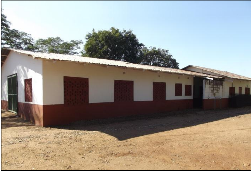
Fig. 26. Site MF 14. Currently used as a fertilizer storage facility, this building served as a military building in the past. It probably approaches 60 years of age.
