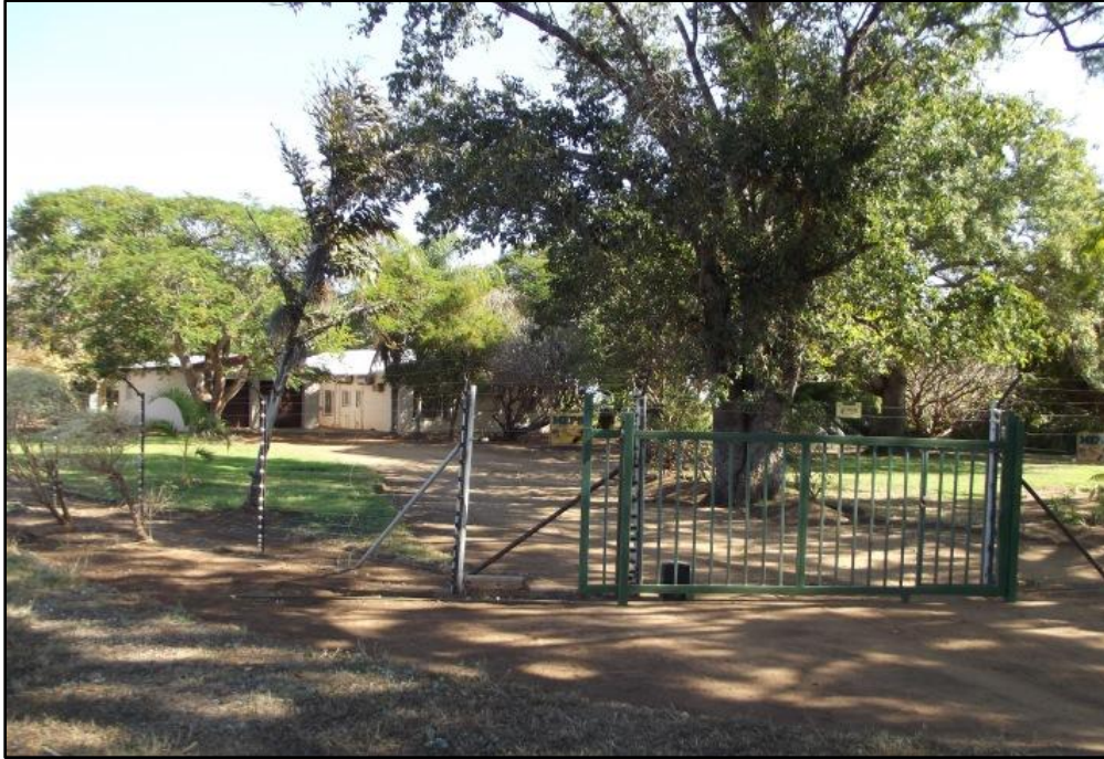
Fig. 24. Site MF 12. Staff housing. Photo taken south-west.
