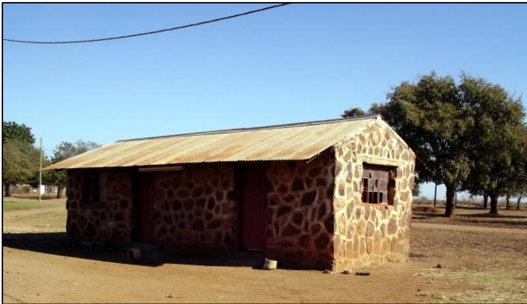
Fig. 39. Site MF 24. Utility shed. Photo taken south.
