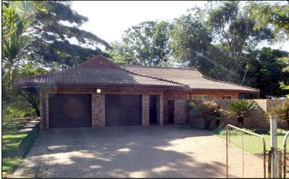
Fig. 34. Site MF 20. Staff residence. Photo taken west.
