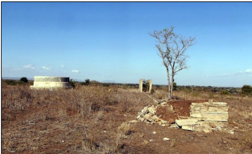
Fig. 19. Site MF 8. The ruined remains of a reservoir. Photo taken in a southern direction.
