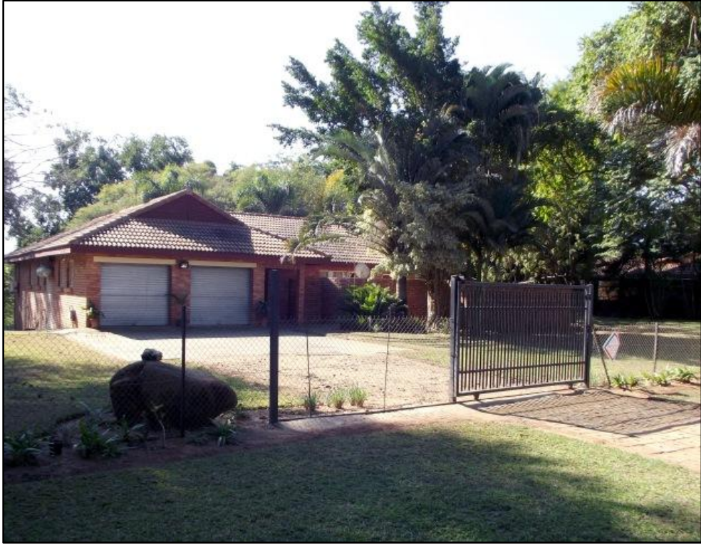
Fig. 28. Site MF 15. Staff residence. Photo taken west.
