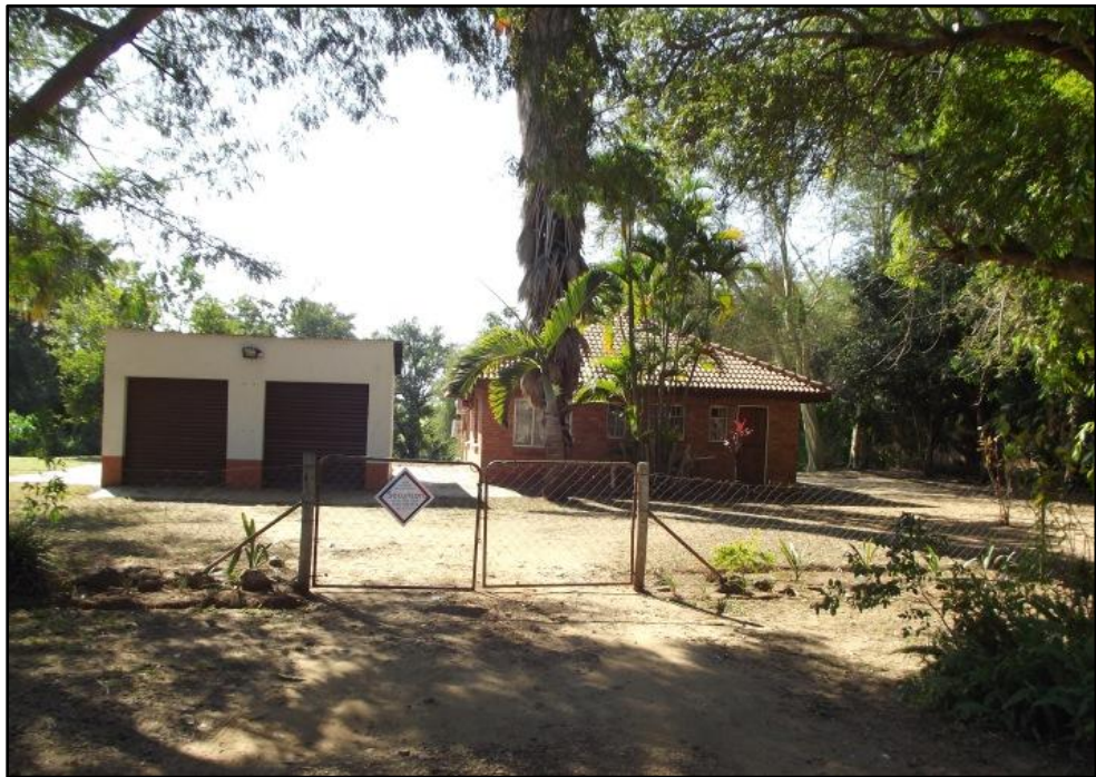
Fig. 29. Site MF 15. Staff residence. Photo taken west.
