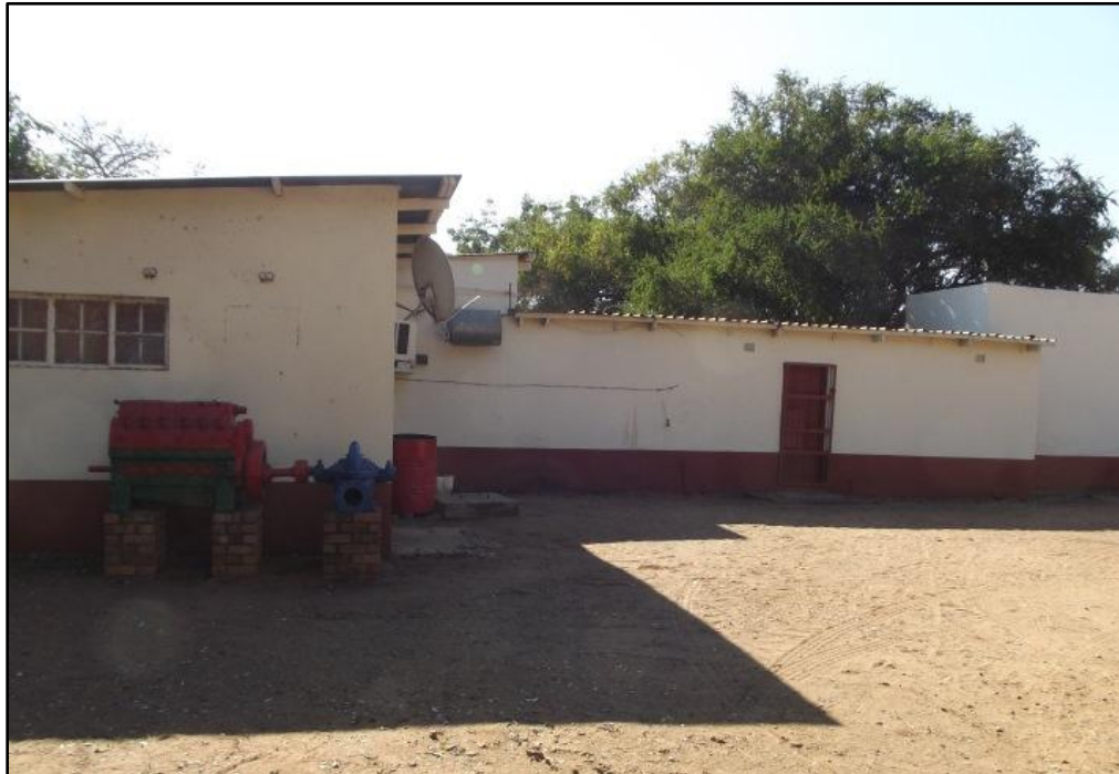
Fig. 27. Site MF 14. A second building which is currently utilized as club house is probably contemporaneous with the current fertiliser storage building.
