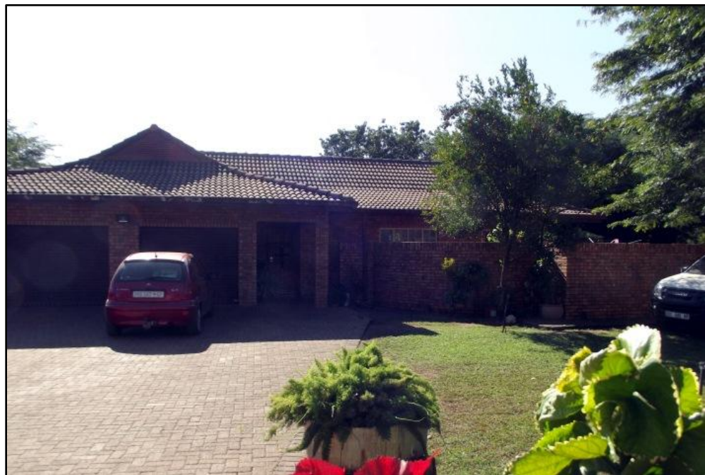
Fig. 35. Site MF 21. Staff residence. Photo taken west.
