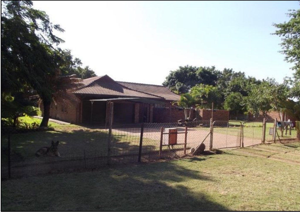
Fig. 32. Site MF 18. Staff residence. Photo taken west.
