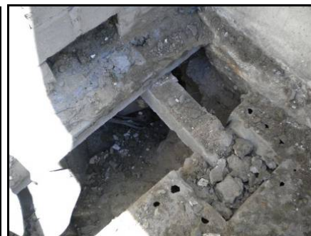
Figure 7: New wall built over lintels.
