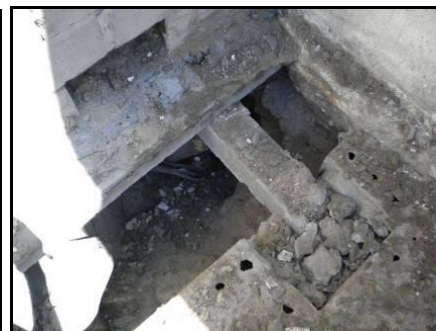
Figure 7: New wall built over lintels.
