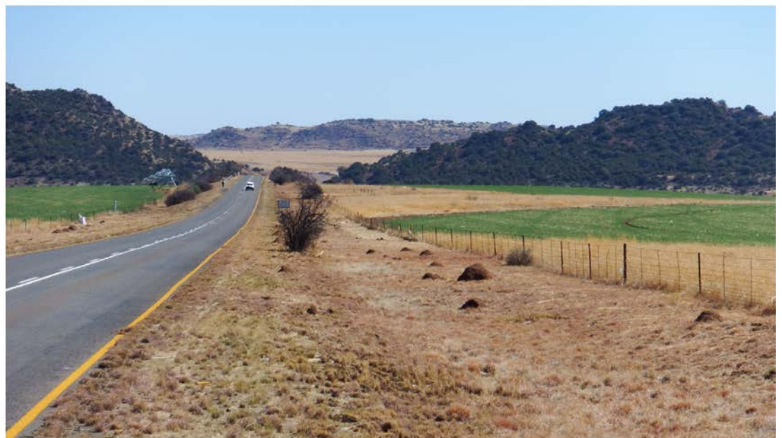
Figure 8. General view of the route along the N6 (top) and secondary tar road (below) between route section points F, G to H.
