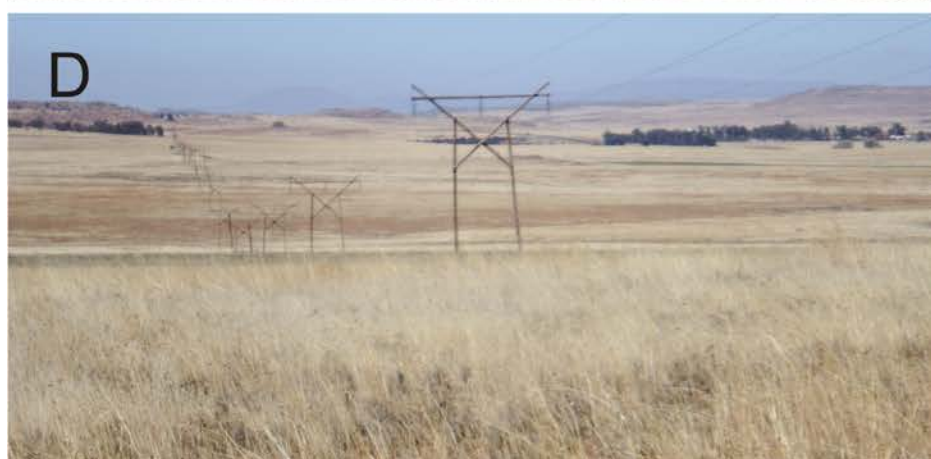
Figure 3. General view of the Rouxville Substation and footprint between route section A-B.
