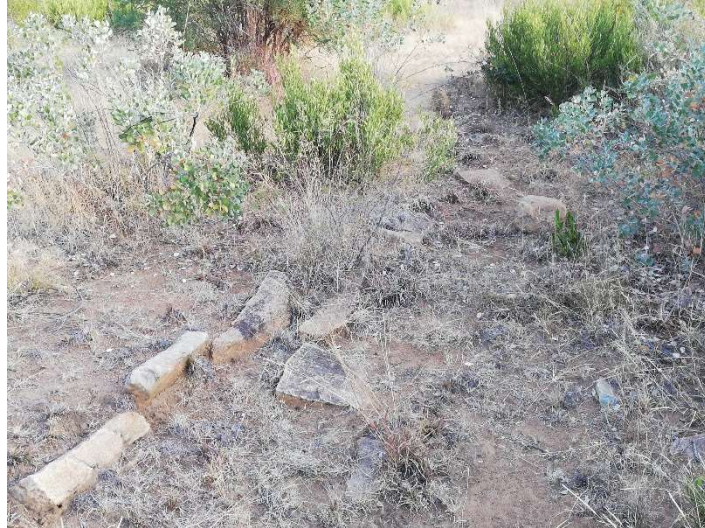
Figure 12: Example of dilapidated linear walling.
