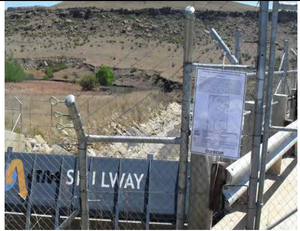
Photo 12: View of the spillway at the intake canal
