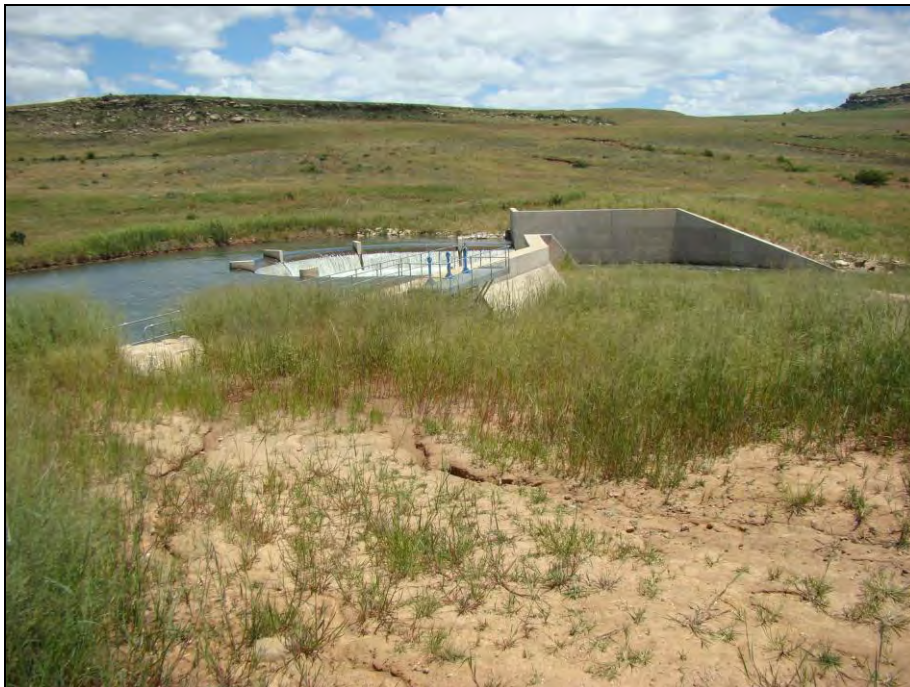
Fig.1 Weir in the Asrivier for hydro-electricity plant at Point A, Marino 1487.
