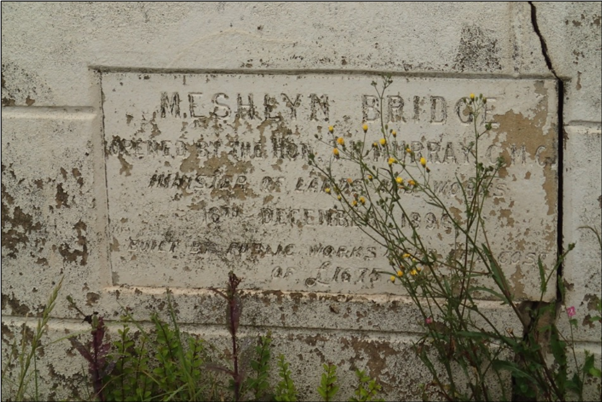
Figure 5. Memorial Plaque on the Meshlyn Bridge
