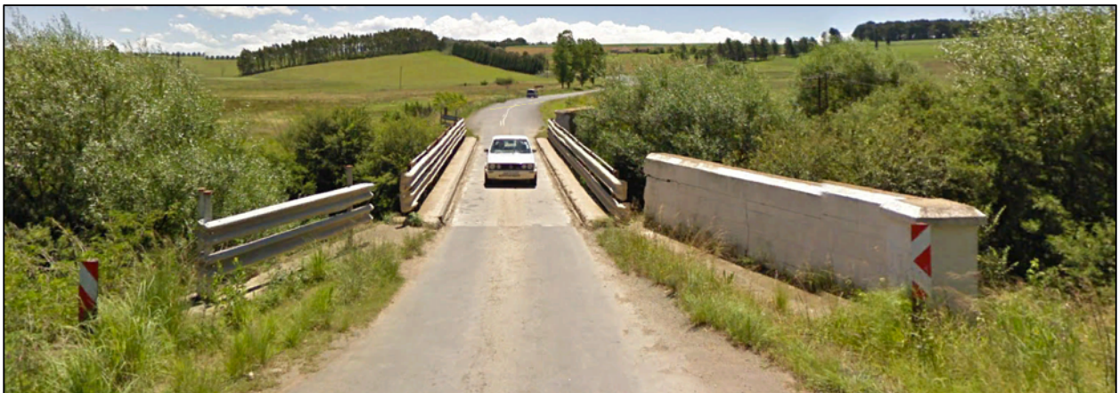
Figure 1. Existing Meshlyn Bridge
