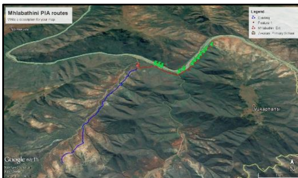
Figure 2 Locality and planning of the Mhlabathini Road Upgrade Project in KZN
