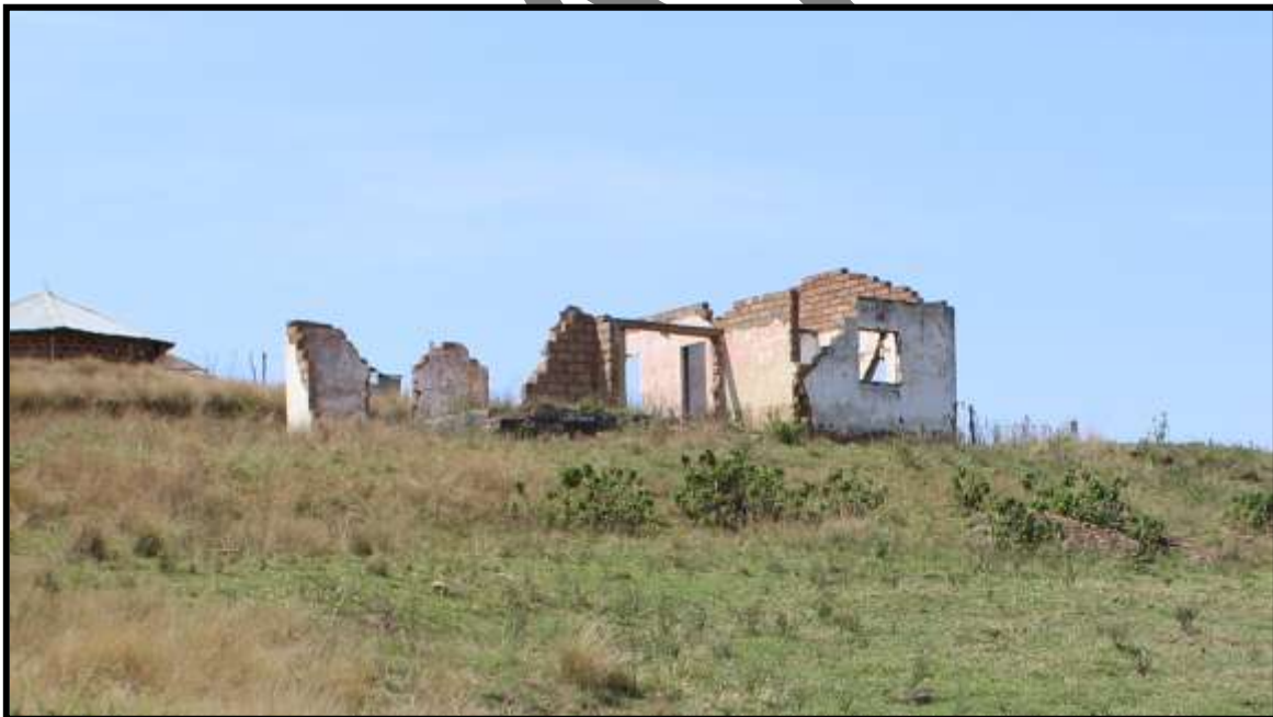
FIG. 15: BUILDING AT HH3
