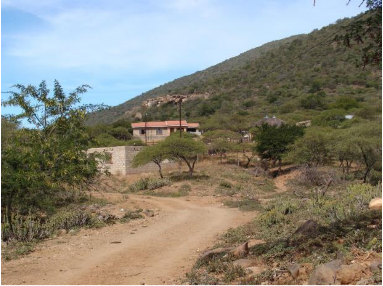
Figure 6: The section of road to be upgraded ends on the slopes of the hillside, corresponding to the blue dot in Figure 1
