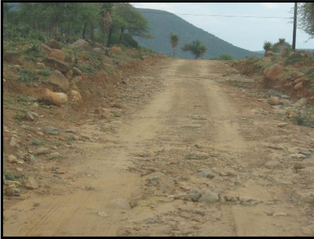
Figure 5. The existing Mhlopeni Mud Track that has been earmarked for upgrading.
